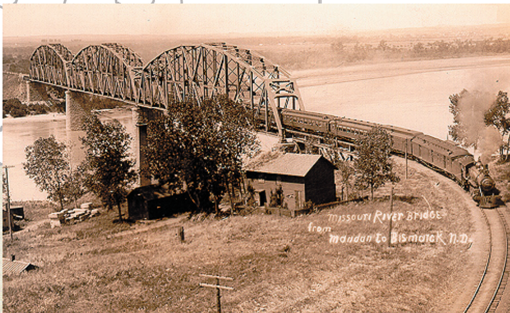
Figure 7: Missouri River Train Bridge from Mandan to Bismarck
