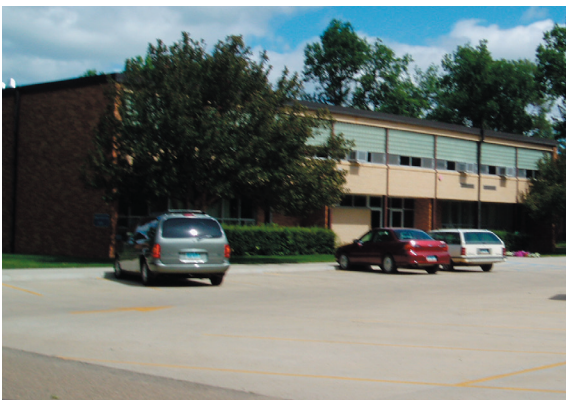
Figure 38: Front of Administration.
