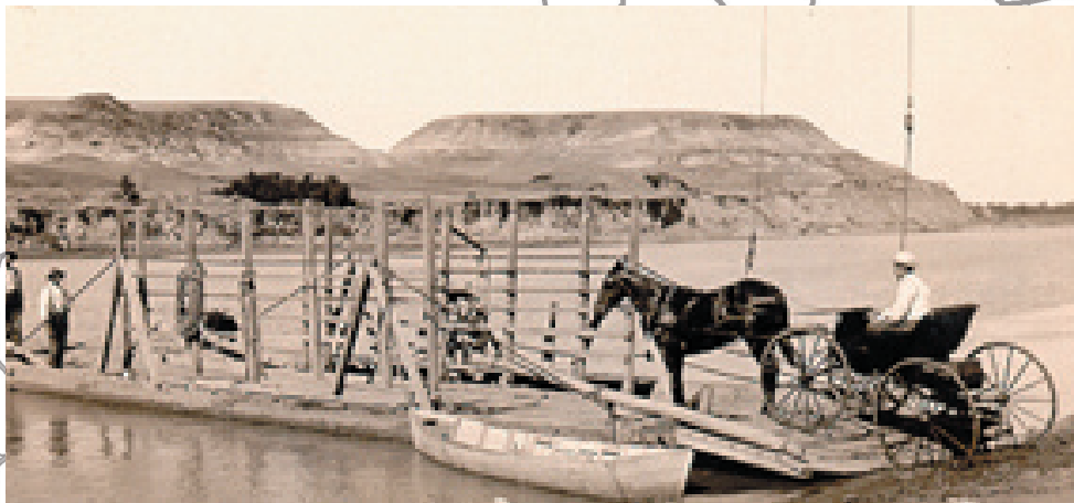
Figure 6: Prior to bridge, forged river with flats
