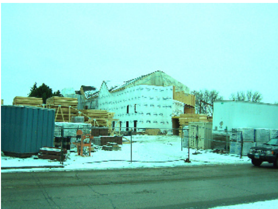
Residential Housing Project Currently Under Construction Located South of Site
