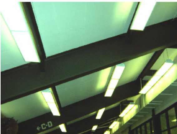
Structure Supporting Second Level Basketball Seating
