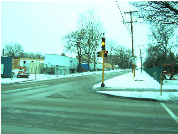
Looking West Down 15th Avenue North
