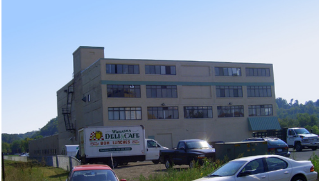
Figure 3.19 - Existing three business building
