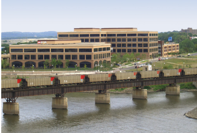
Figure 3.16 - Existing US Bank building
