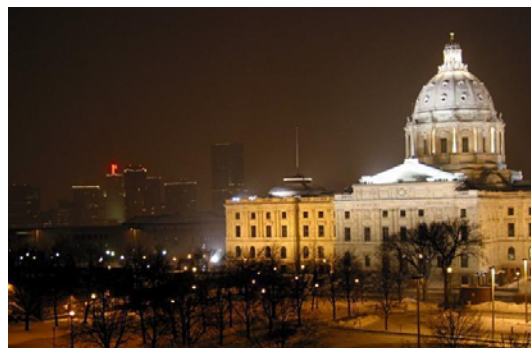
Figure 3.28 Minnesota State Capitol Building
