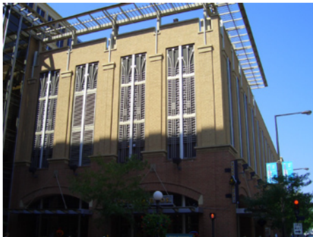
Figure 3.10 - Existing Parking Structure
