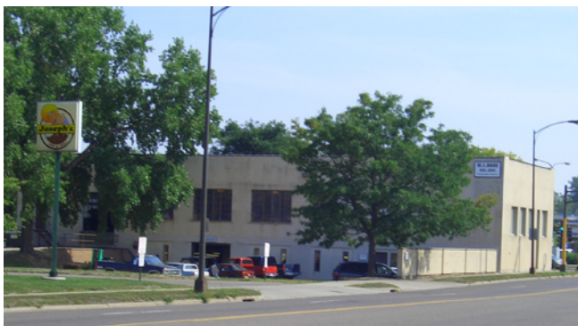
Figure 3.20 - Existing W.I. Maas Mfg. Corp.
