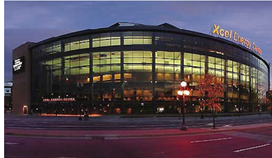
Figure 3.26 The Xcel Energy Center
