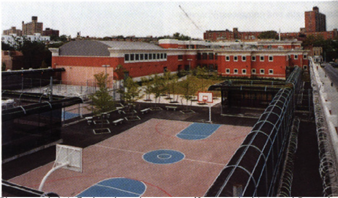
Photograph 1.4 Enclosed outdoor space (Source: Architectural Record 12-1998)
