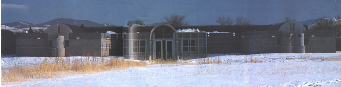
Photograph 1.5 Exterior of center
