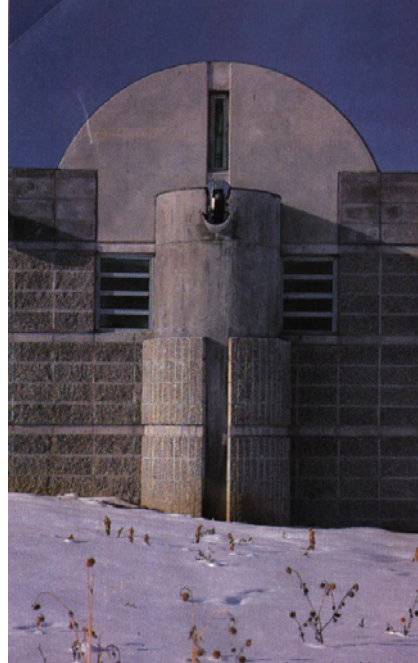
Photograph 1.7 Roof Vaults (Source: Architectural Record 3-1983)
