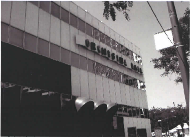
north facade close up
