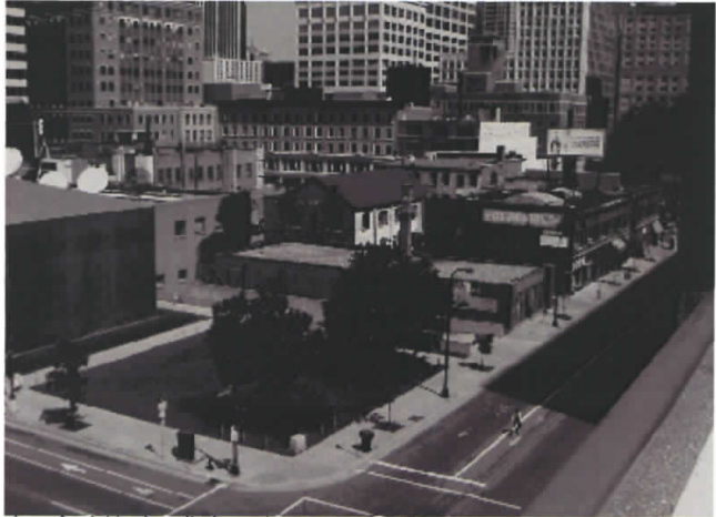
view of neighboring site from above
