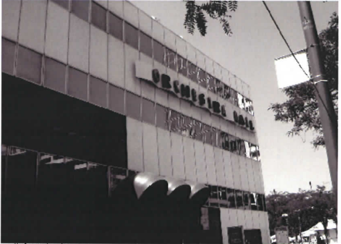
north facade close up
