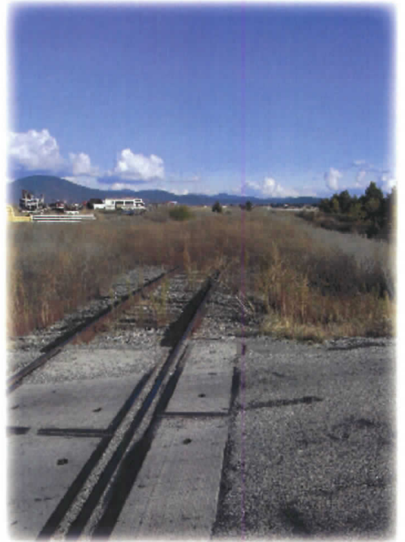
Southeast View - Railroad Tracks
