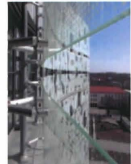
The atrium areas have been protected by a combination of both pendent and sidewall nozzles, insuring adequate window protection.
