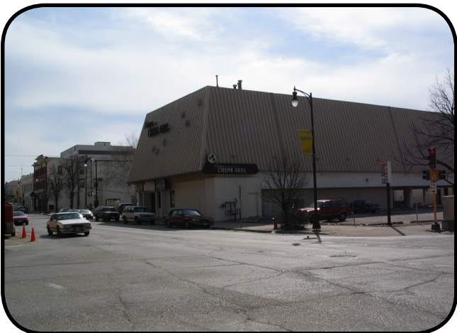
Opposite North East Corner Looking South
