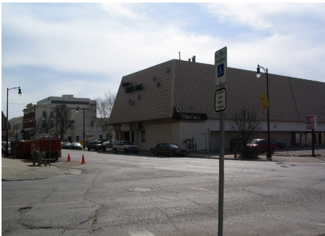
Opposite North East Corner Looking Southeast
