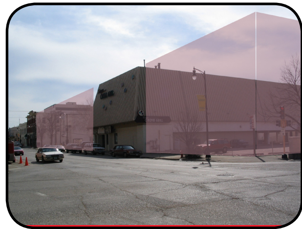
Northeast Corner Looking East
