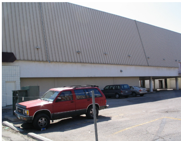
Opposite North East Corner Looking Southeast
