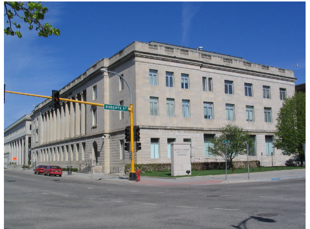
Northwest Corner Looking Northwest
