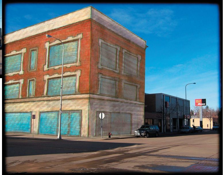
Renovation at the Corner of 1st St N and 1st Ave W Proposed Main Level Retail and Upper Level Residential
