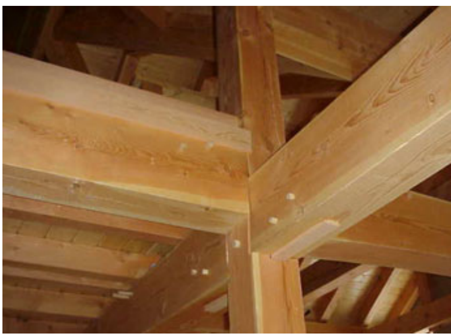
Mortise and Tenon Timber Frame
