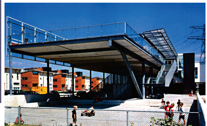
Terrace cantilevering out over the play area with the row houses in the background.
