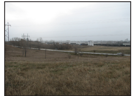
Northeast - Fall 2005 Enbridge above ground storage tanks
