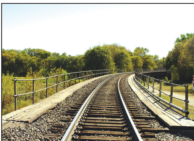
The BNSF Railroad Bridge
