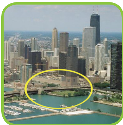
Figure 1.10. North-West View of Site
