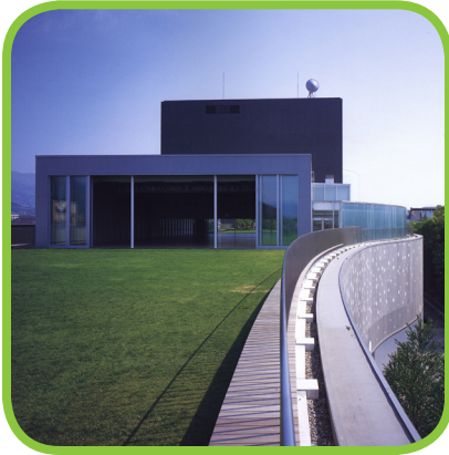
Fig.2.62. Green Roof Terrace
