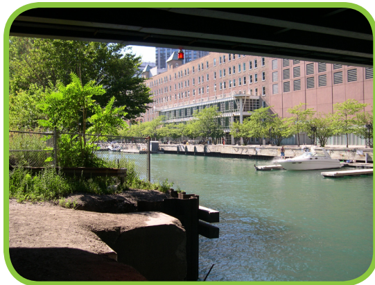
Fig.4.37. Under Lake Shore Bridge looking west
