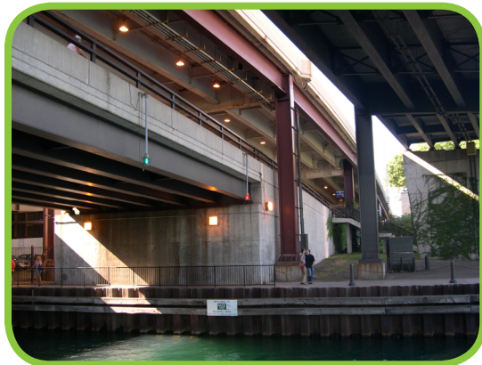
Fig.4.38. Under Lake Shore Bridge looking North
