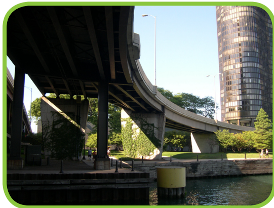
Fig.4.39. Under Lake Shore Bridge looking North
