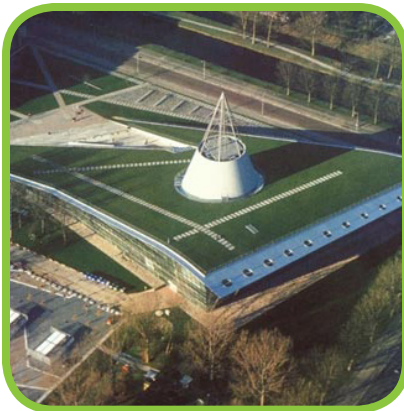
Fig.2.58 Aerial showing Green Roof
