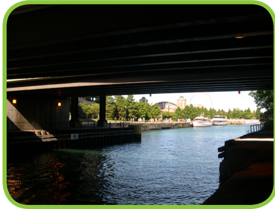
Fig.4.36. Under Lake Shore Bridge looking east
