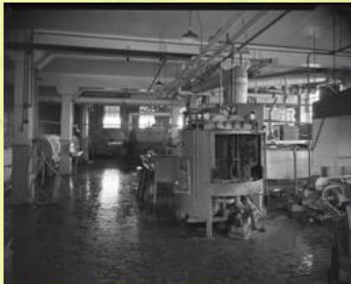
Basement Armour Creamery Building
