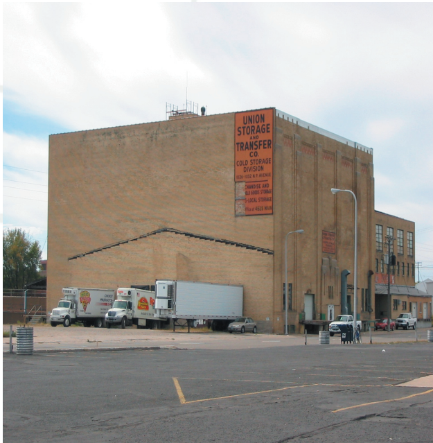
East Side of Building
