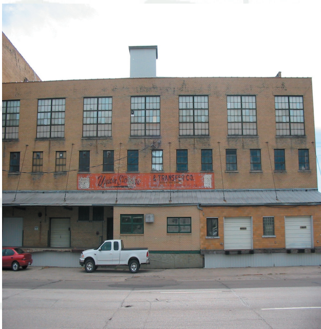
North Side of Building - West Half
