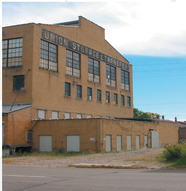
West Side of Building
