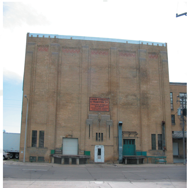
North Side of Building - East Half
