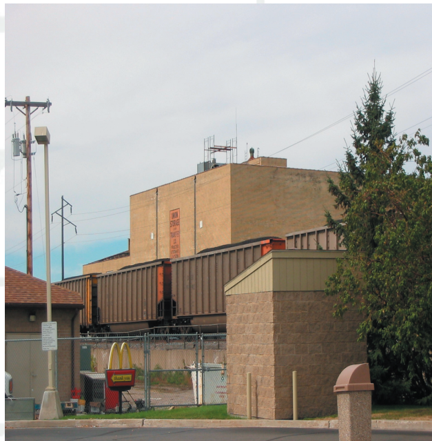
South East Side of Building
