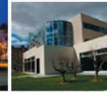
LIBRARY AND LECTURE HALL ENTRANCE
