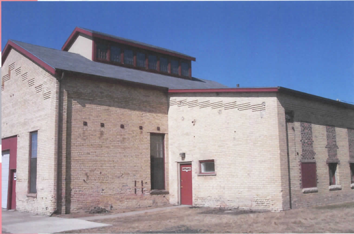
Engine House Building: No 7
