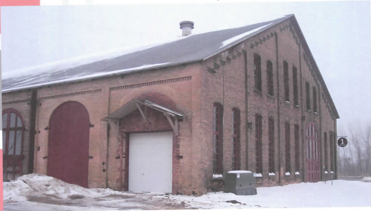
Boiler Shop Building: No1
