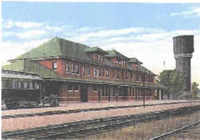
Northern Pacific Depot Building. Brainerd, Minnesota. Dated 1928. Washington Street (HWY 210).
