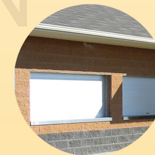
Concession Stand and Announcer Booth -Salmon and Slate Split Face Concrete Blocks
