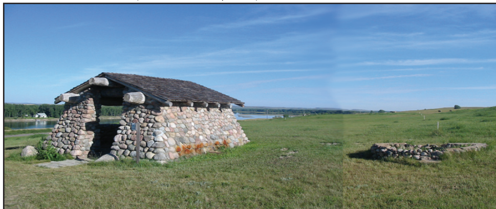
fig.2-10 CCC Shelter West Side of Site (Personal Photo, 2005) .
