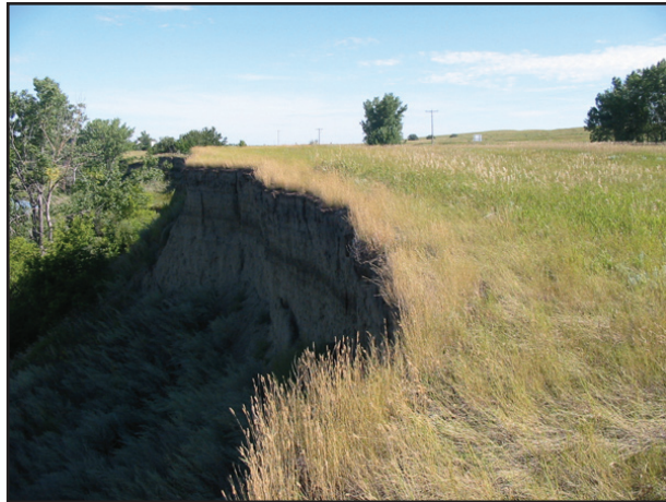
fig.2-16 North Adjacent Property (Personal Photo, 2005).
