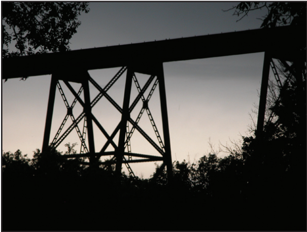
fig.2-85 Valley City High Line Bridge Hansen, et al. 2005.
