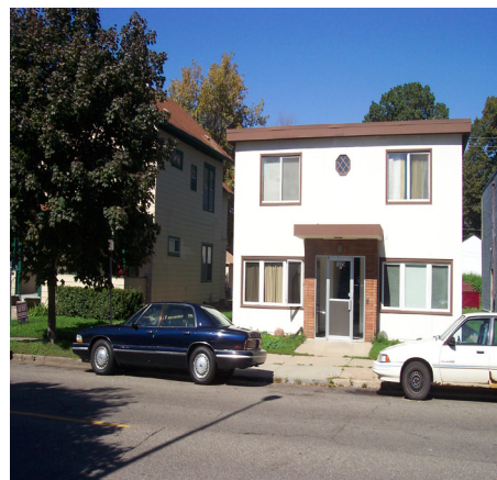
view west showing apartments of theatre
