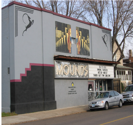
view looking at south facade
