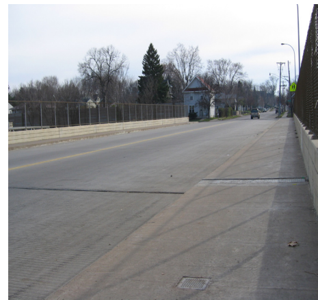
view looking south on bridge over I94
