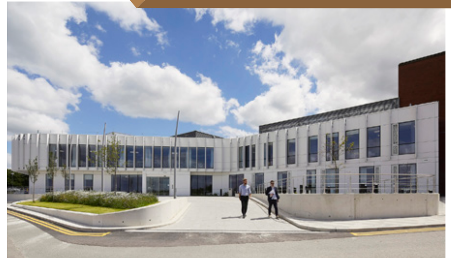
NORTHWEST - MAIN ENTRANCE
