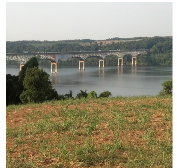
Figure 39 | Millard E. Tydings Memorial Bridge
