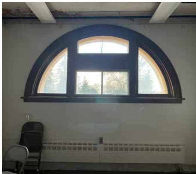
Figure 23 - Window on first floor of the central main tower
