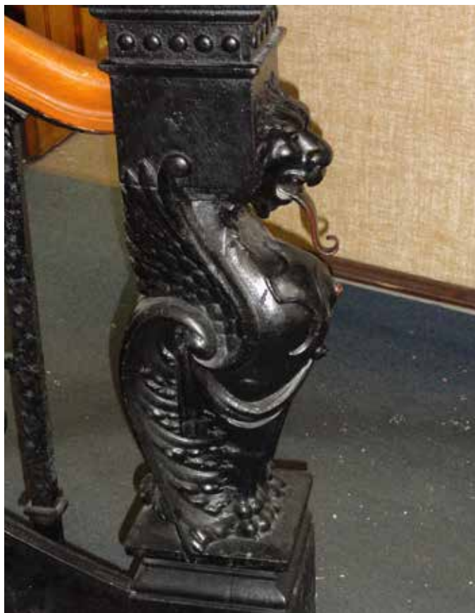
Figure 27 - Grand staircase railing detail
