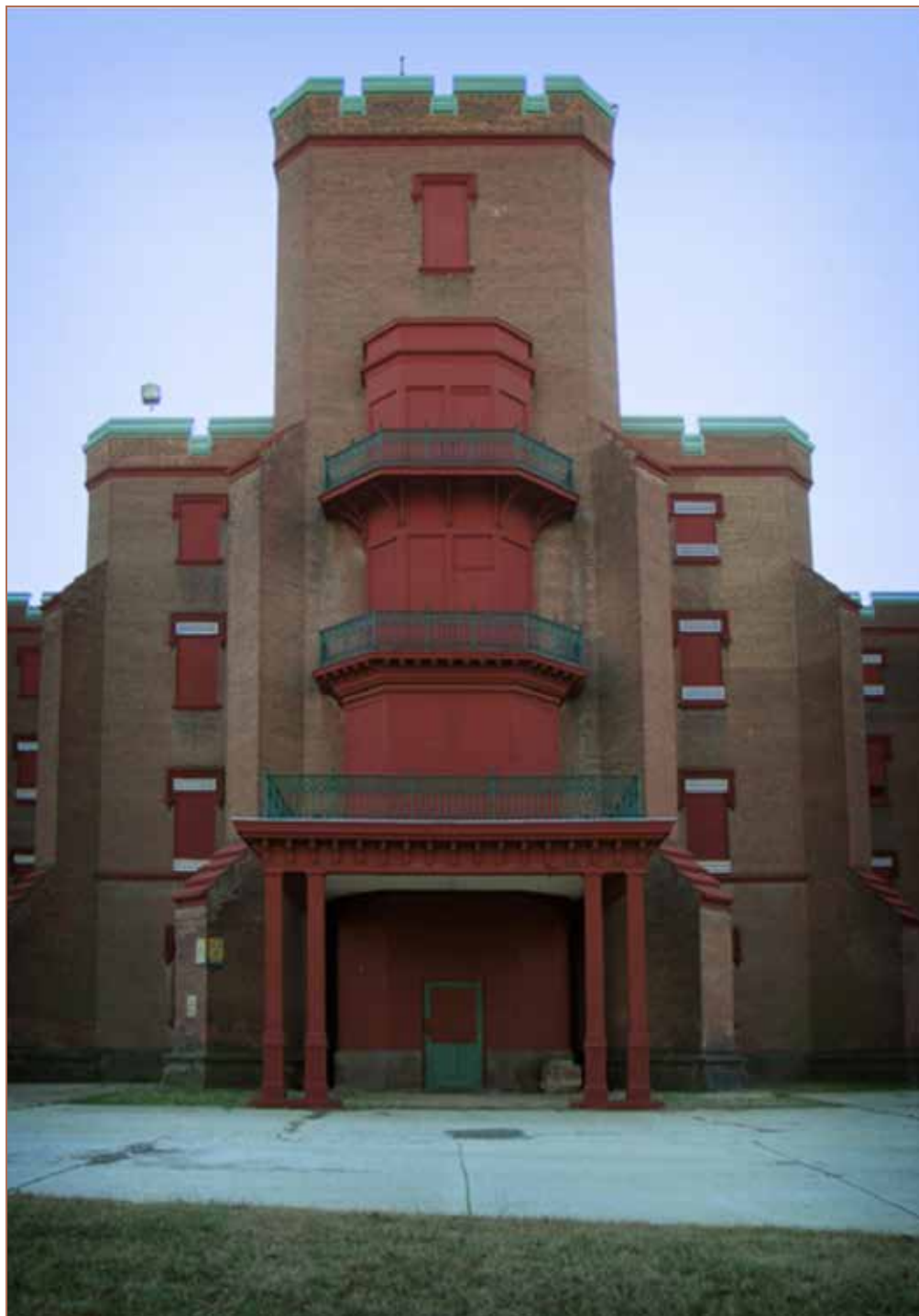
Figure 11 - St. Elizabeth's Hospital Central Tower
