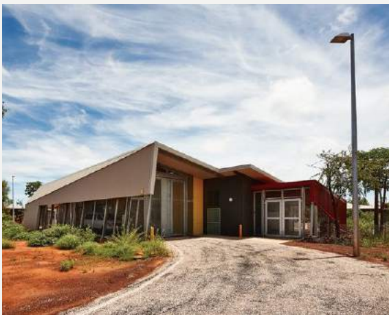
Figure 163—Kimberley Services Building (from West Kimberley Regional Facility)
