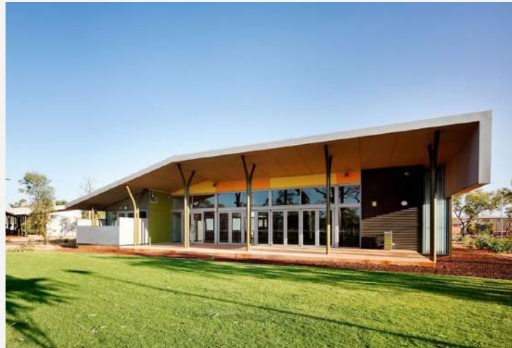
Figure 162—Kimberley Programs Building (from West Kimberley Regional Facility)
