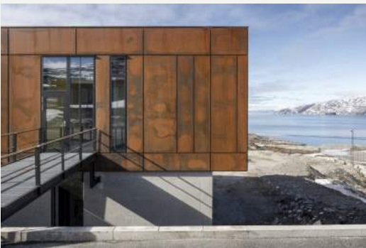
Figure 139—Burnt Sienna Facade (from SHL)
