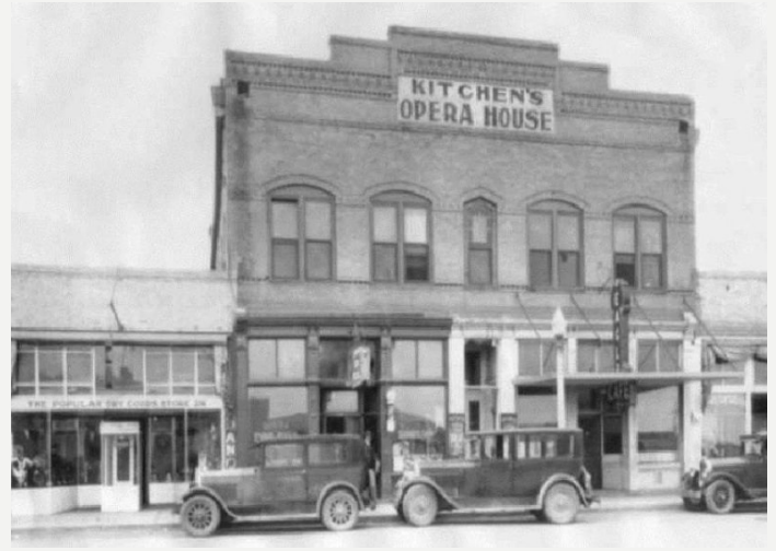
Figure 96—Kitchens Opera House 1920 (from Preserve America)
