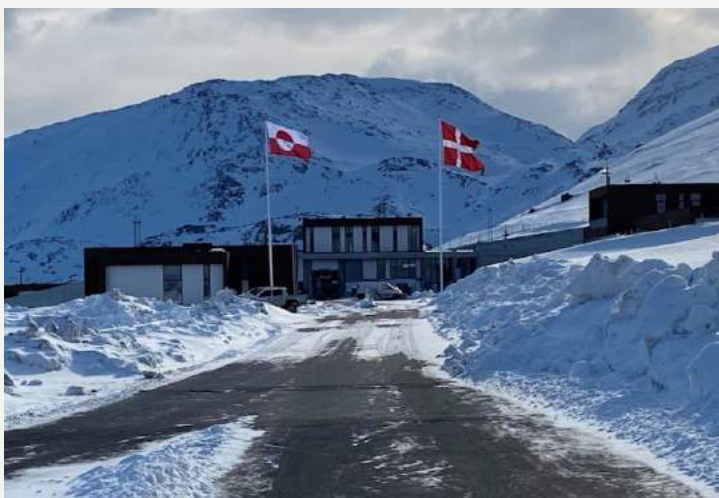
Figure 137 —Anstalten Entrance (from Cold Comfort )
