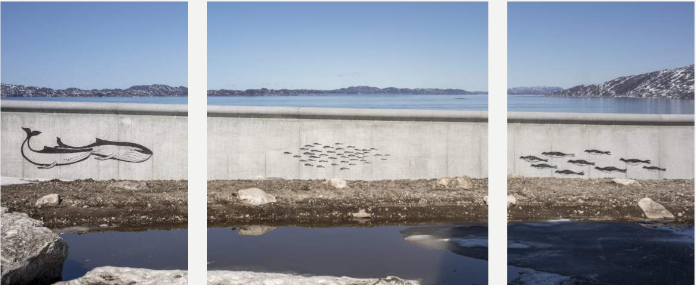
Figure 145—Anstalten Perimeter Wall (from SHL Anstalten Correctional Facility)
