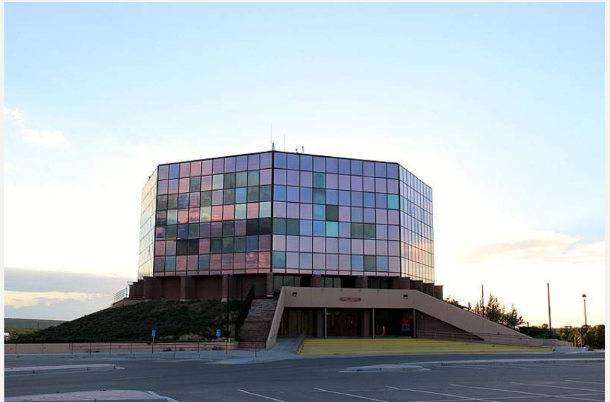
Figure 108 —Ned A Hataali Center at Diné College (from Diné College)
