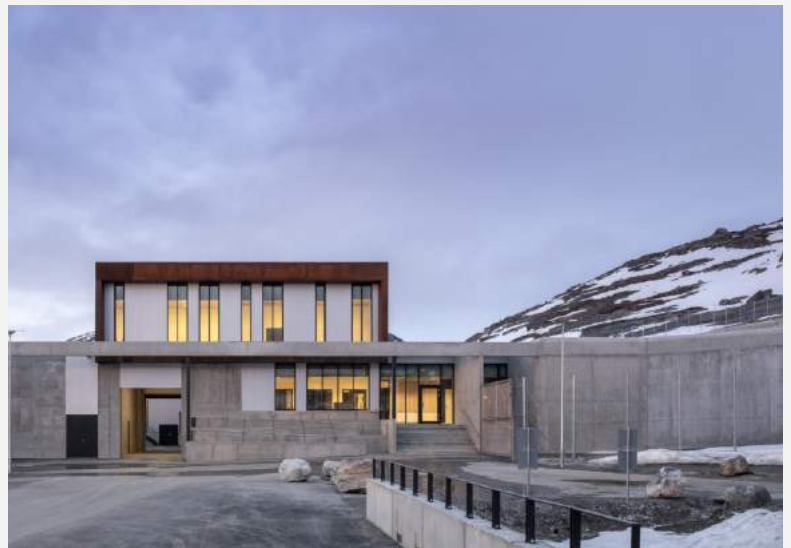
Figure 141—Anstalten Perspective (from SHL Anstalten Correctional Facility)
