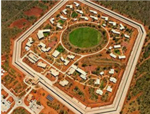
Kimberley Aerial View (from ABC Local Australia)
