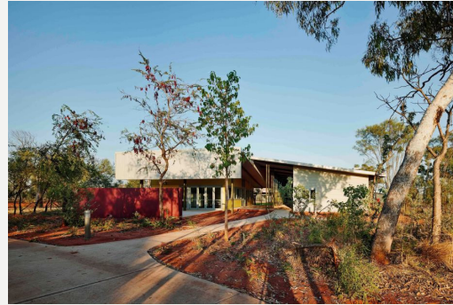
Kimberley Housing Building 1 (from West Kimberley Regional Facility)
