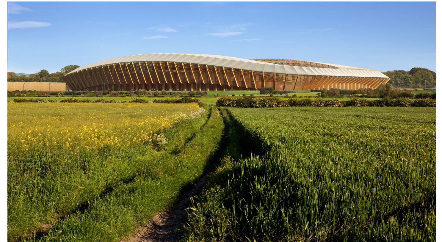
Fig. 57 Eco Park Stadium
