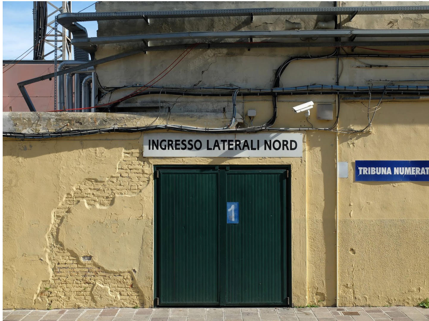
Fig. 72 Existing Stadium North Entrance
