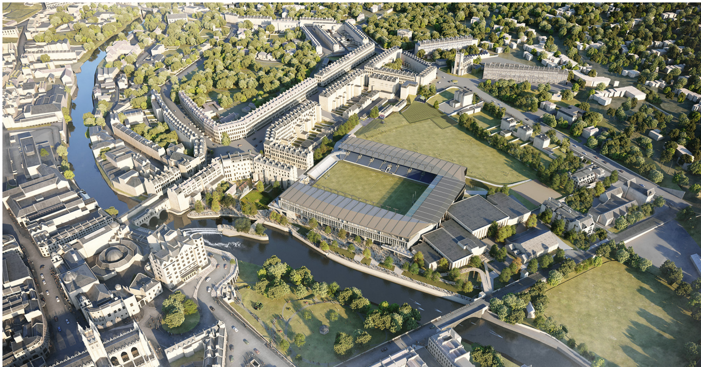
Fig. 48 Bath Rugby Stadium site
