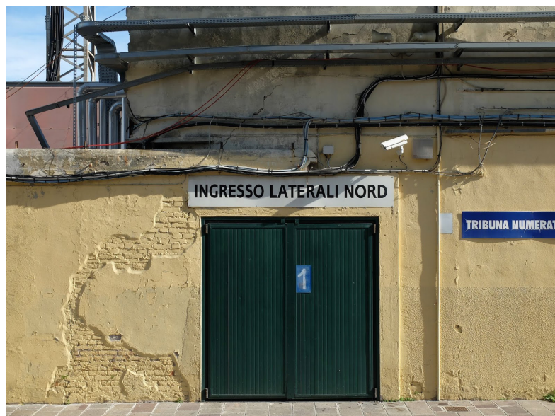
EXISTING NORTH ENTRANCE
