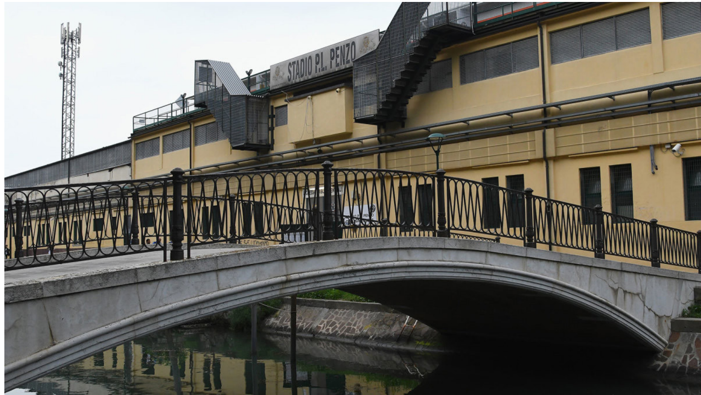
Fig. 75 Existing Pedestrian Bridge and Main Entrance
