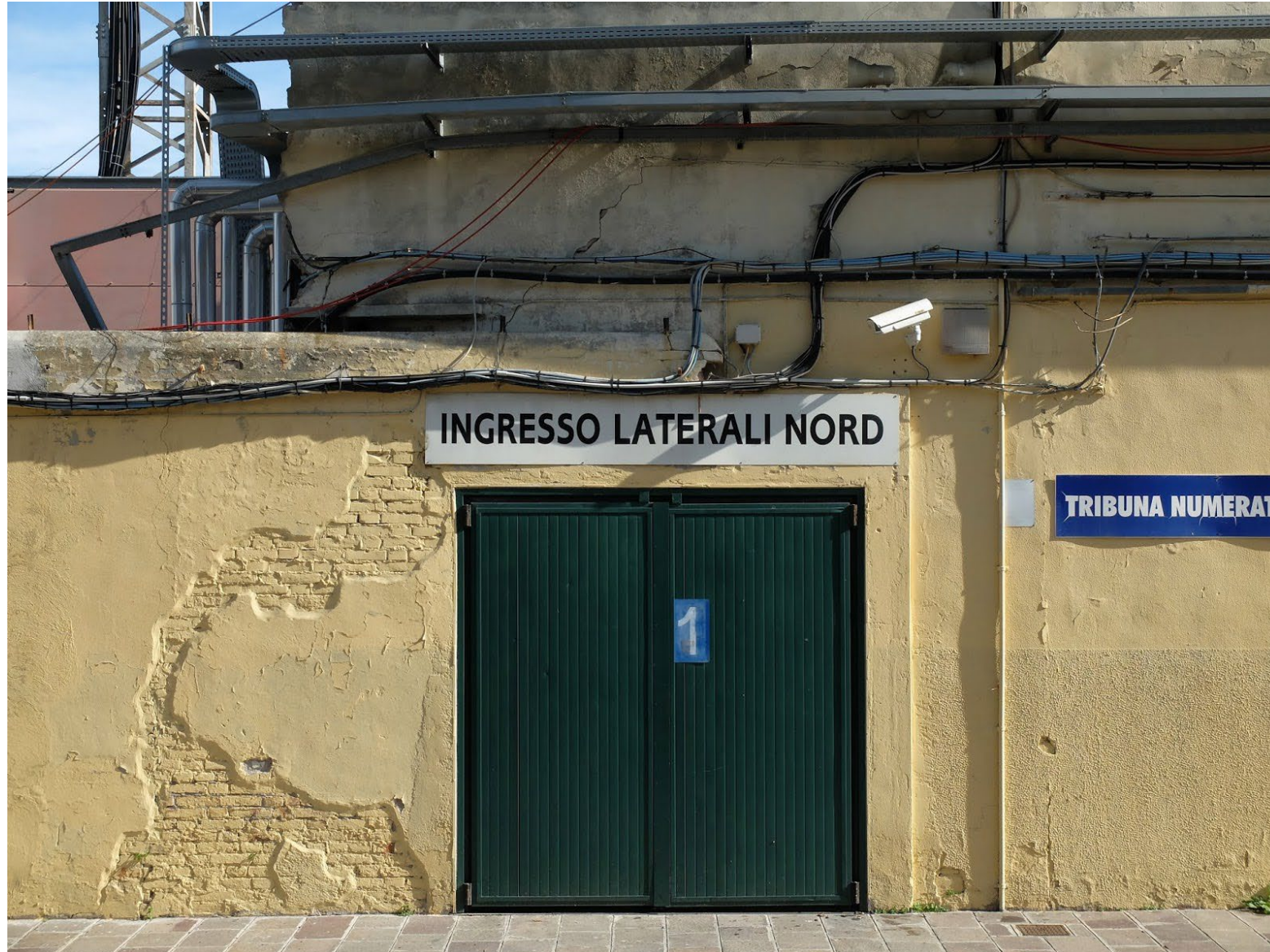
EXISTING NORTH ENTRANCE
