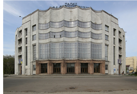
ORIGINAL FRONT ENTRANCE
