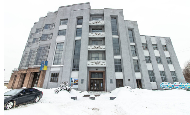
SIDE ENTRANCE- EAST VIEW
