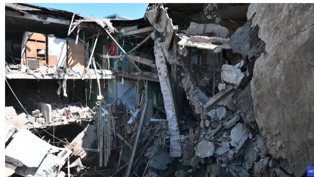
INTERIOR NOW EXPOSED
