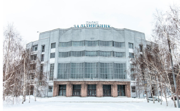
MAIN ENTRANCE- SOUTH EAST VIEW
