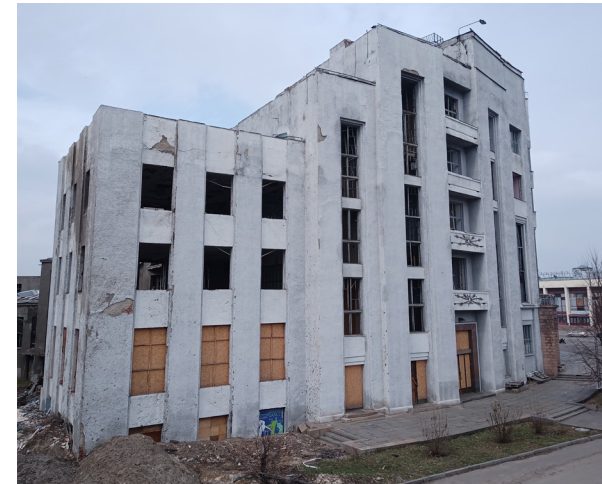
SOUTH ENTRANCE AFTER SHELLING SHOWING EXTERIOR SHELL INTACT
