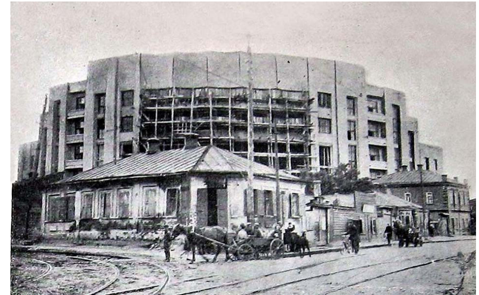
PALACE OF CULTURE FOR RAILWAY WORKERS DURING CONSTRUCTION
