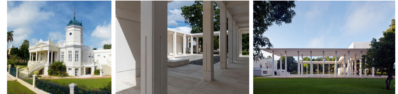
FRONT ENTRANCE TERRACE PORTICOES
