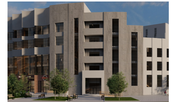
REBUILT EAST ENTRANCE
