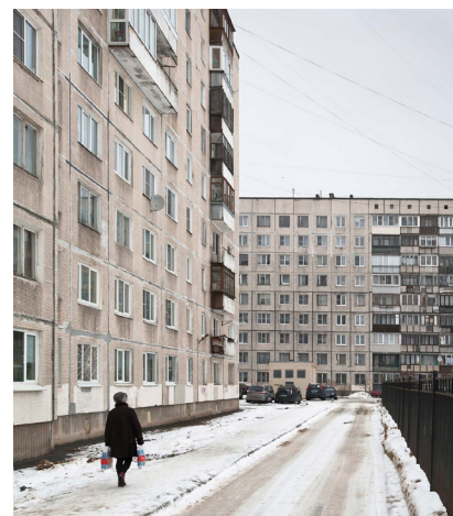
PRE-FAB PANEL APARTMENT BUILDING
