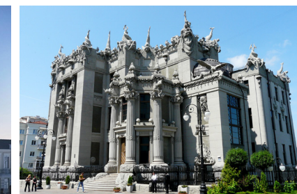
THE HOUSE WITH CHIMAERAS, KYIV, UA
