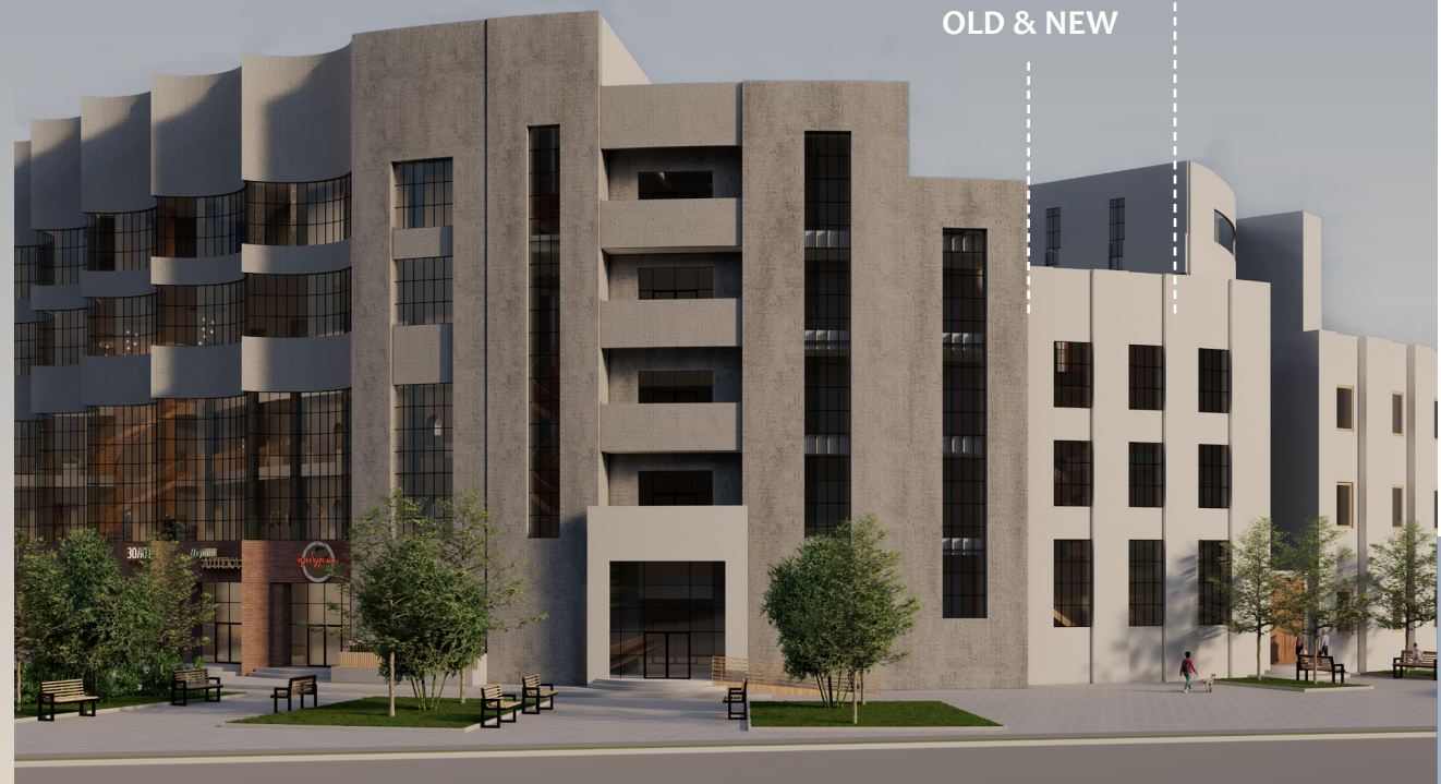
EAST ENTRANCE SHOWING NEW AND OLD PORTIONS
