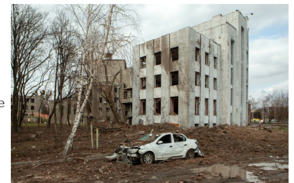
DESTROYED PALACE OF CULTURE FOR RAILWAY WORKERS IN KHARKIV
