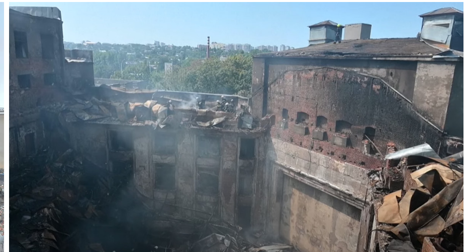
AUDITORIUM AFTER SHELLING
