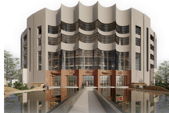
REBUILT FRONT ENTRANCE
