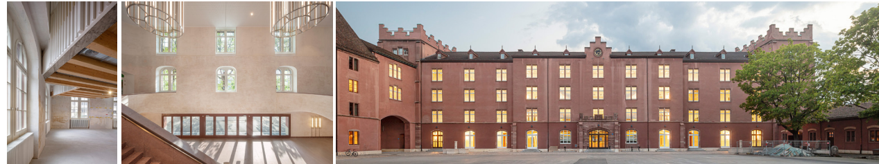
NEW AND OLD MATERIALS MEET ENTRY ATRIUM FRONT ENTRANCE AND PLAZA
