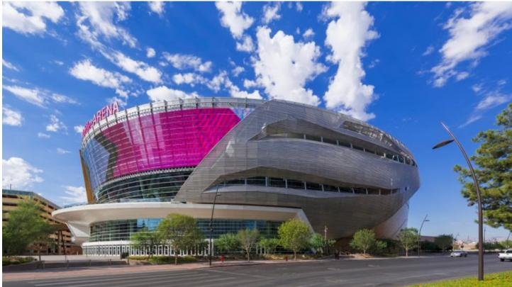
Primarily, T-Mobile Arena is constructed of structural steel with composite concrete floors. This design features a long span roof which covers the 350 foot by 450 foot seating bowl with no help from columns giving spectators unobstructed views. An expansive rigging grid is capable of supporting 2 Boeing 737 airplanes, or 180,000 pounds.
