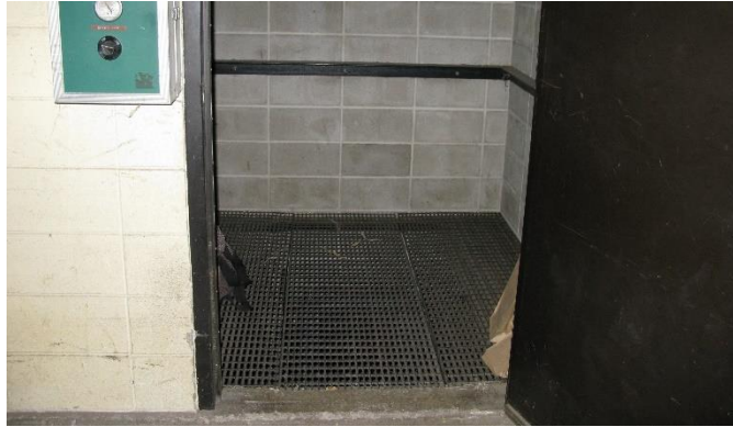
Figure 19. Purpose built drying rooms consist of a perforated floor, a heat source, and a fan. Heated air is blown up through the floor; the air temperature and flow rate can be controlled.
