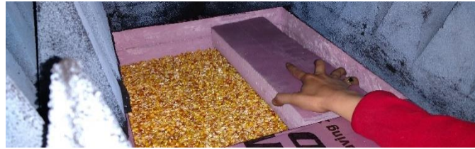
Figure 10. Granular material is smoothed/leveled by hand
