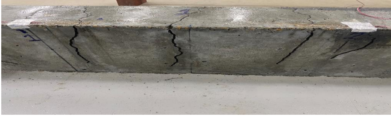
Figure 34. Cracks for Sample 1 after the Test
