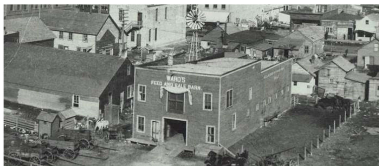
One of Rugby's Oldest Surviving Buildings (1907)
