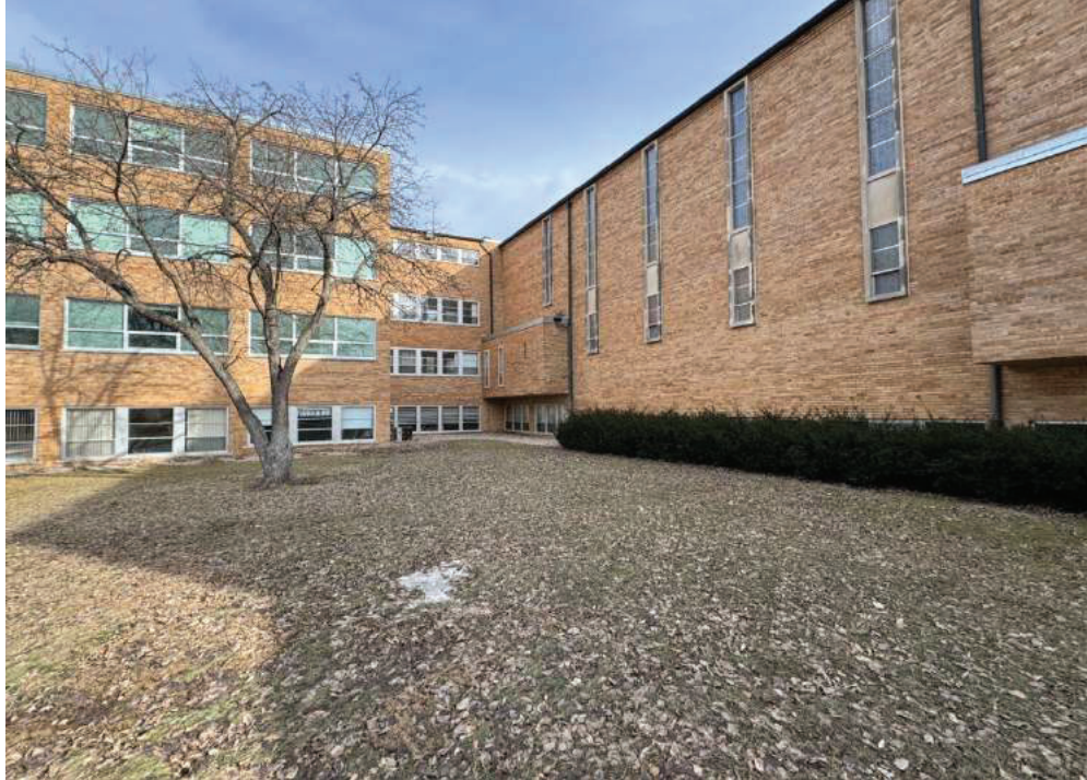
Figure 48 North end of convent (left) and chapel (right)
