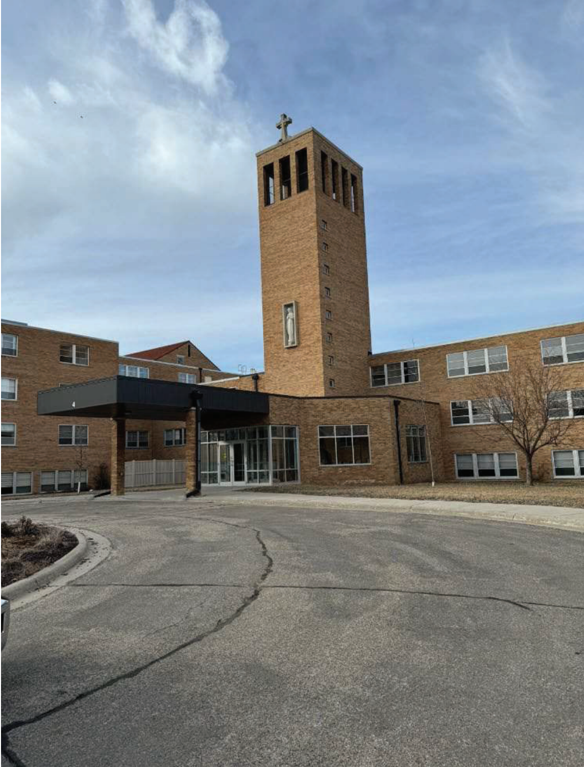
Figure 45 South entrance of administration building
