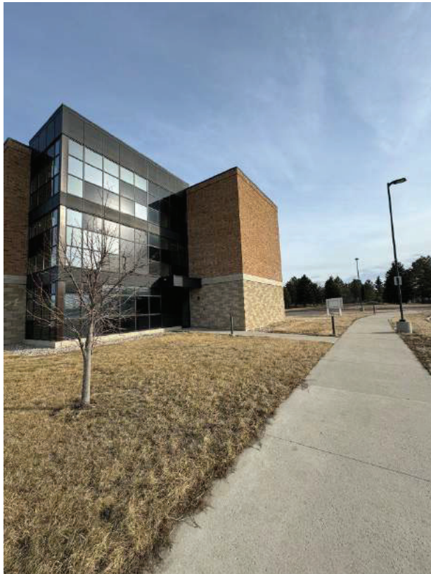
Figure 54 West entrance of east student housing suites
