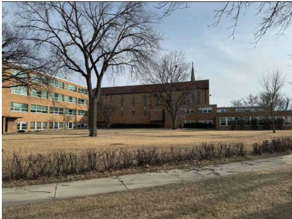
Figure 47 North end of convent (left), chapel (center), priest quarters and mechanical and boiler area (right)
