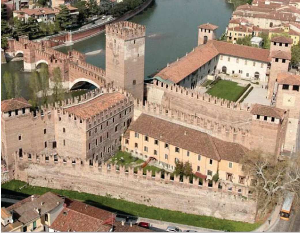
Figure 7 The Castelvecchio Museum in Verona, Italy, as shown above, was worked on by Carlo Sarpa from 1957 to 1974.
