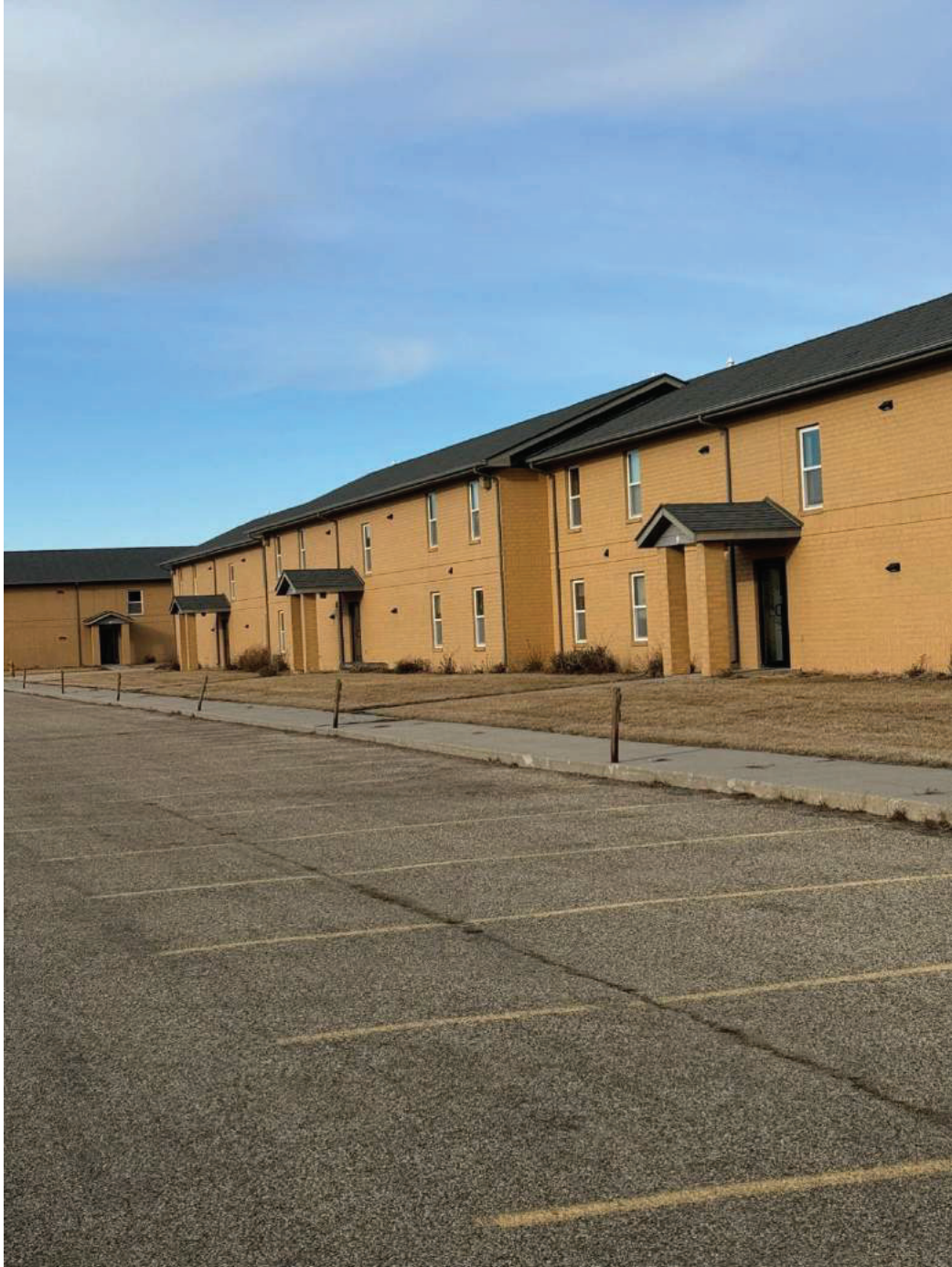
Figure 57 West façade of north student housing complex building
