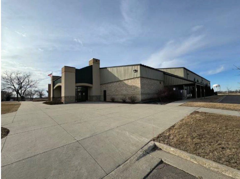
Figure 58 Strode Activity's Center (built 1998)
