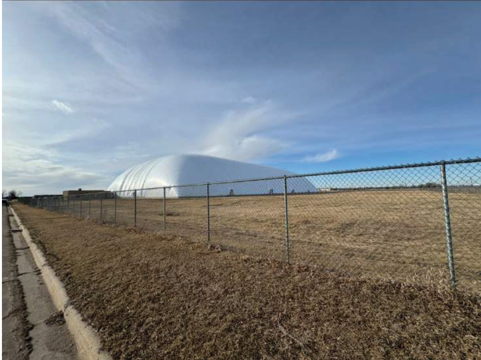
Figure 62 Southwestern facade of Winter Dome
