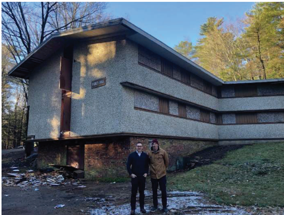
Figure 98 Fobes Hall, one of the last three remaining dorms of Nasson College to be redeveloped.
