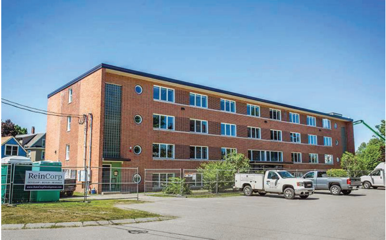
Figure 97 Former Maryland Hall for Nasson College redeveloped into senior housing. Source: MaineBiz
