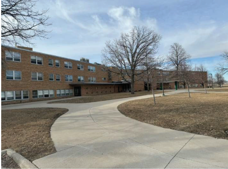
Figure 43 East entrance of administration building (built 1993)
