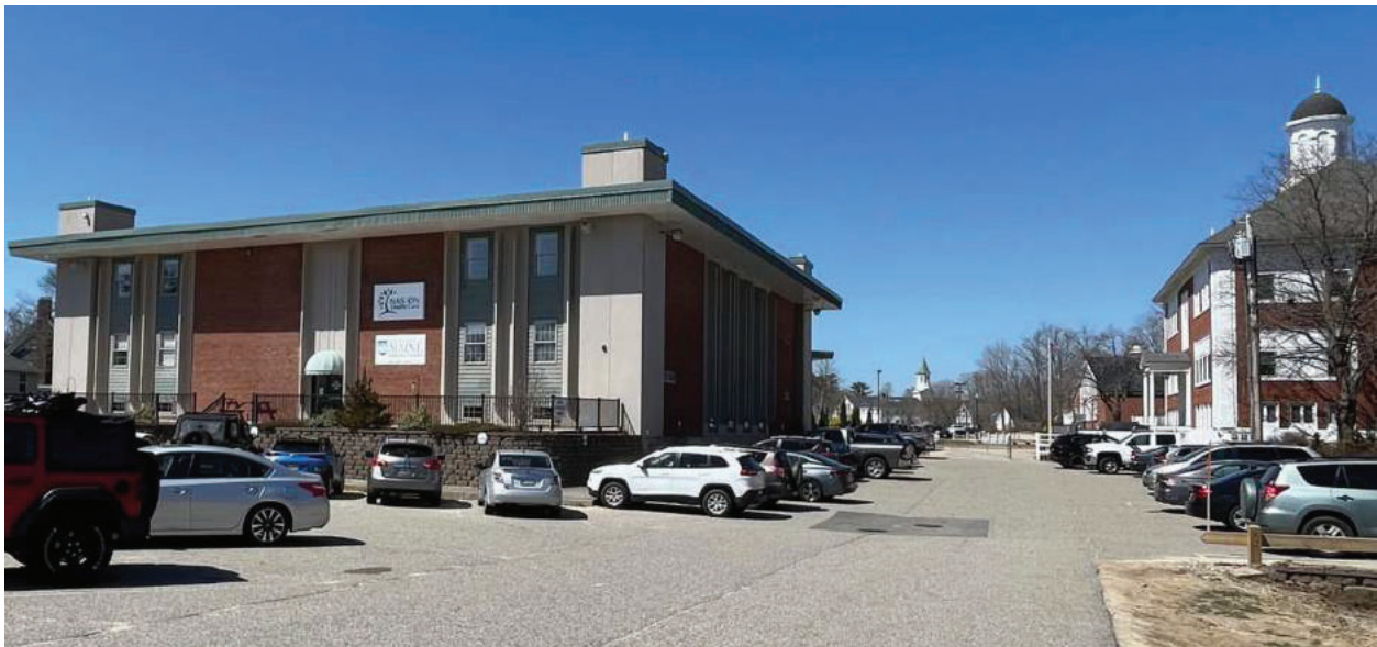
Figure 96 The original science building was repurposed into a community health center in 2012 with tenants Nason Health Care, a division of the York County Community Action Corporation, and NorDx Maine Health.
