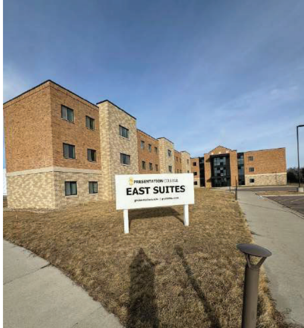
Figure 53 East student housing suites (built 2013)
