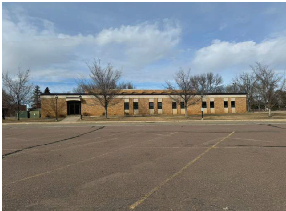
Figure 52 West exterior of Nurse's Education Building
