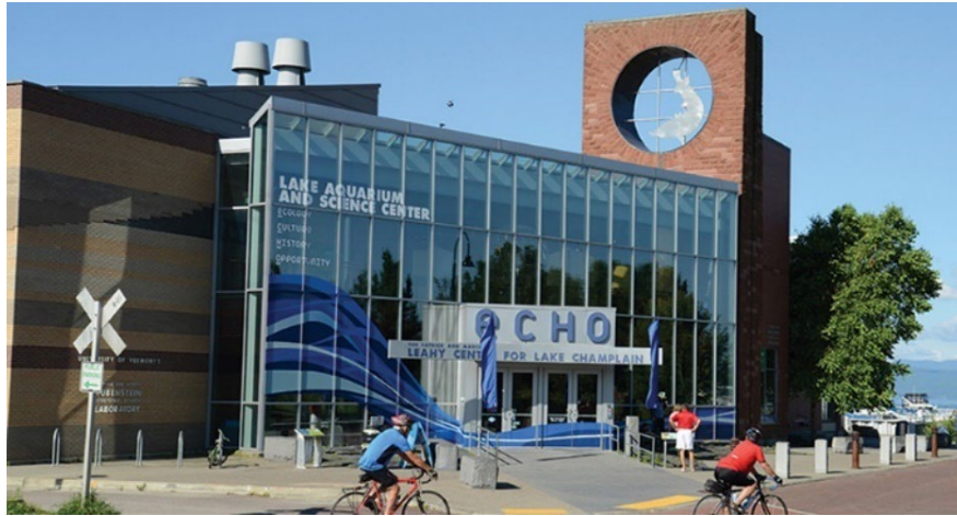
Figure 20. ECHO Front Entrance
