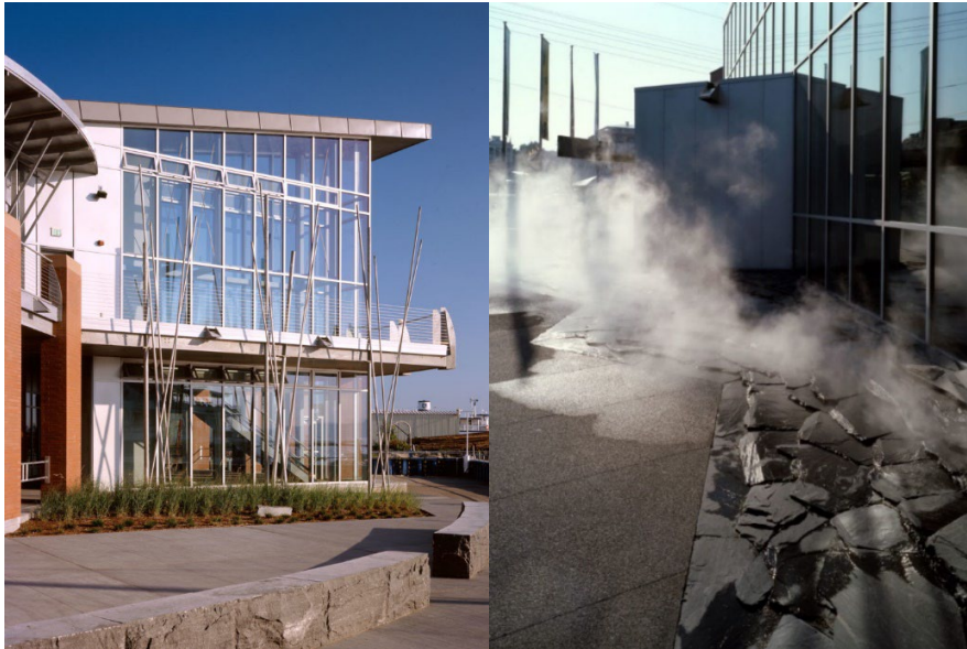
Figure 38. ECHO Leahy Center Site Features
