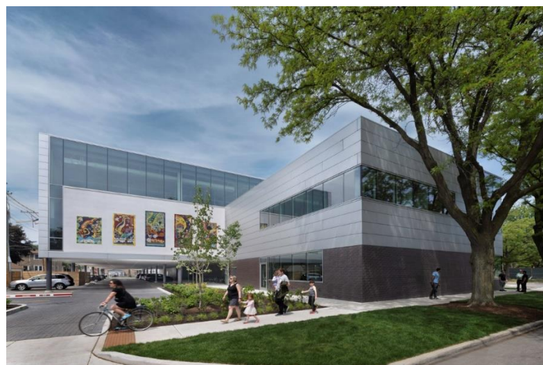
Figure 57. OPCRC Exterior Façade (from Oak Park Community Recreation Center / Perkins&Will, 2023 )
