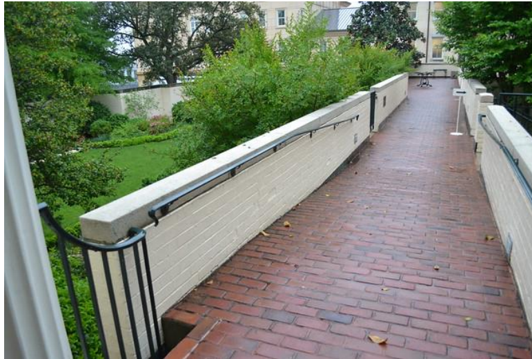
Figure 3. Accessible Ramp at Federal Building (from Paralyzed Veterans of America , 2023)
