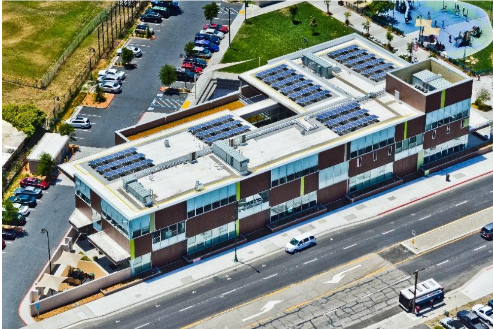
Figure 47. Exterior view of the building. Roof showing the solar panels on REACH Ashland Youth Center designed by RDC Architecture Inc. (Architizer, 2013). https://architizer.com/projects/reach-ashland-youth-center/
