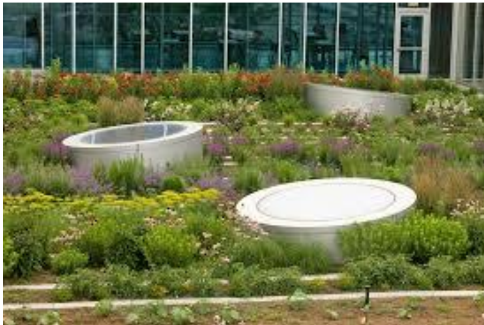
Figure 66. View of skylights on the green roof. Gary Comer Youth Center was designed by John Ronan Architects in 2006. (HoerrSchaudt, 2006). https://hoerrschaudt.com/project/gary-comer-youth-center/
