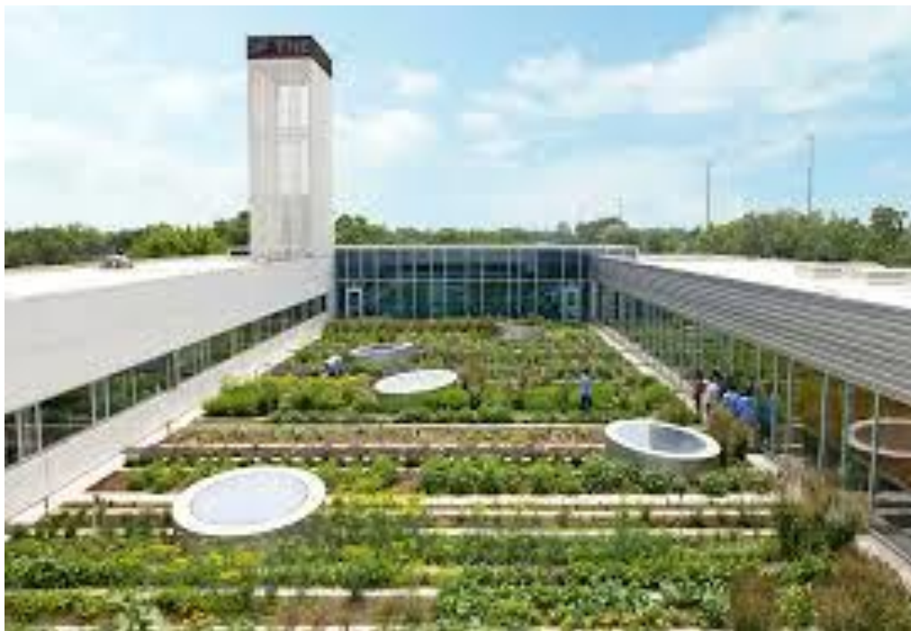
Figure 64. View of the green roof, skylights, and the walls of glass that connect the roof with the rest of building. Gary Comer Youth Center designed by John Ronan Architects in 2006. (HoerrSchaudt, 2006). https://hoerschaudt.com/project/gary-comer-youth-center/
