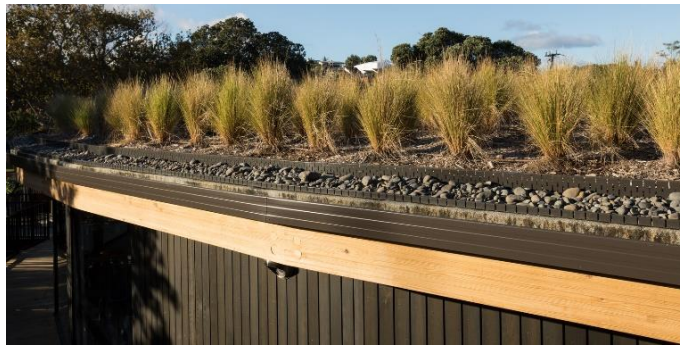
Figure 34. Close up of the different levels that make up the green roof. Smith Architect's 2022 Kakapo Creek Children's Garden. (Scowen, 2022). https://www.markscowen.co.nz/kakapo-creek-childrens-garden
