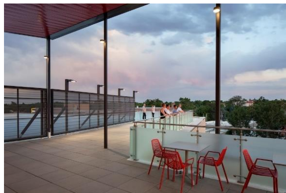
Figure 91. View of the rooftop event space. Carla Madison Recreation Center designed by BRS Architects in 2018. (Spahn, 2018). https://pkelectrical.com/portfolio_post/carla-madison-central-denver-rec-center-denver-colorado/
