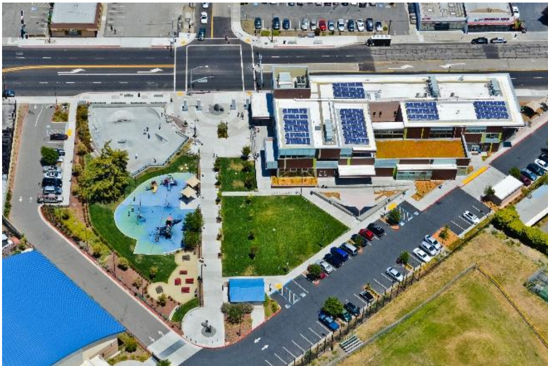
Figure 46. Site plan of REACH Ashland Youth Center designed by RDC Architecture Inc. (Architizer, 2013). https://architizer.com/projects/reach-ashland-youth-center/
