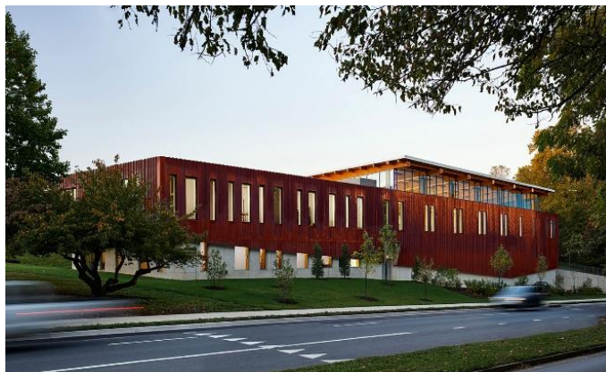
Figure 77. Exterior view of the Lubber Run Community Center from the street to the North. (VMDO Architects, 2020). https://www.vmdo.com/lubber-run-community-center.html
