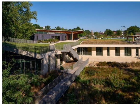
Figure 74. Exterior view of the building showing the ground and green roof connection. Lubber Run Community Center. (VMDO Architects, 2020). https://www.vmdo.com/lubber-run-community-center.html
