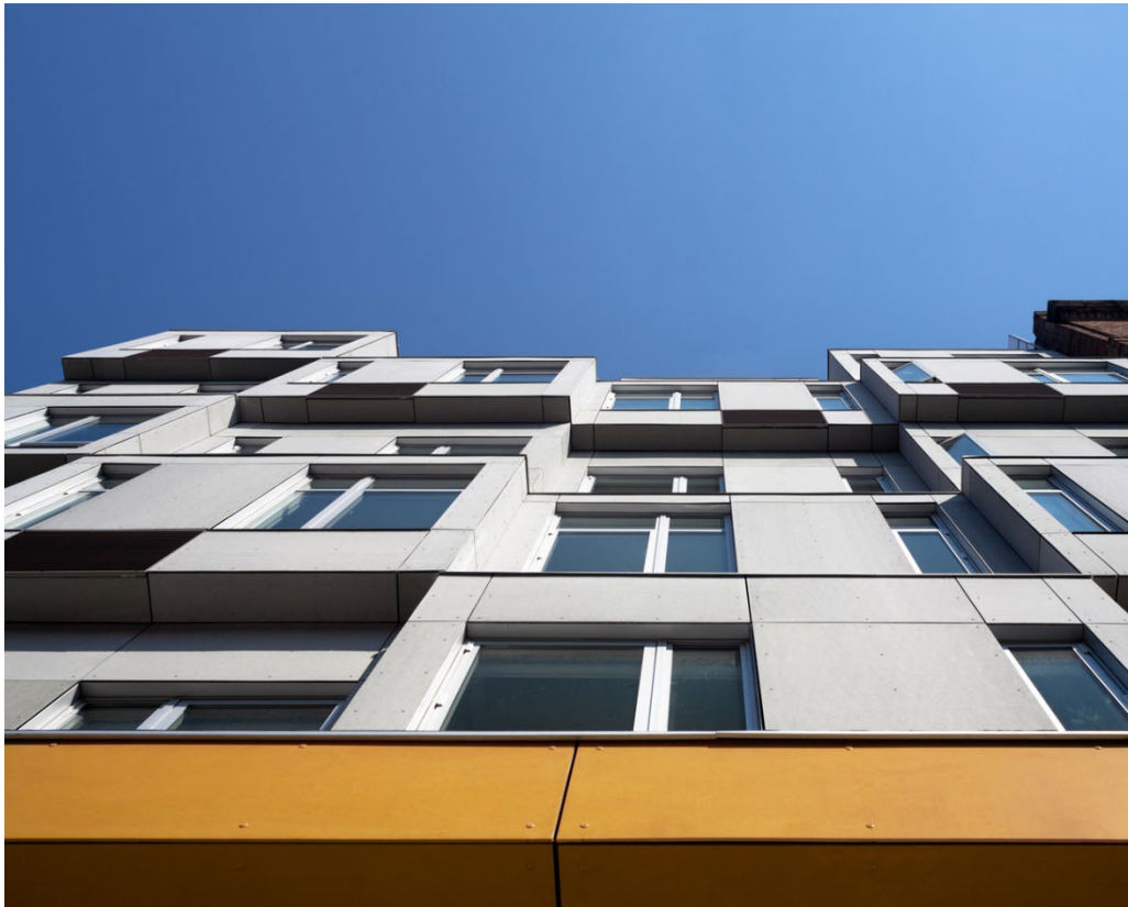
Figure 44. Photograph detailing the “push and pull” notion of the front exterior façade giving light to the modular anatomy of the complex. Credit: Amy Barkow / GLUCK+
