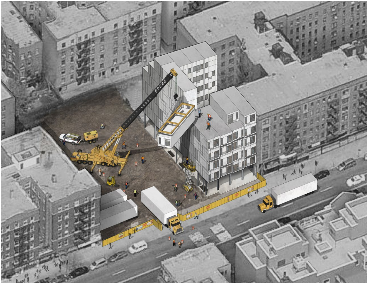
Figure 51. Image that illustrates the construction process of The Stack NYC with the assemblage of the individual modules into one building. Credit: GLUCK+
