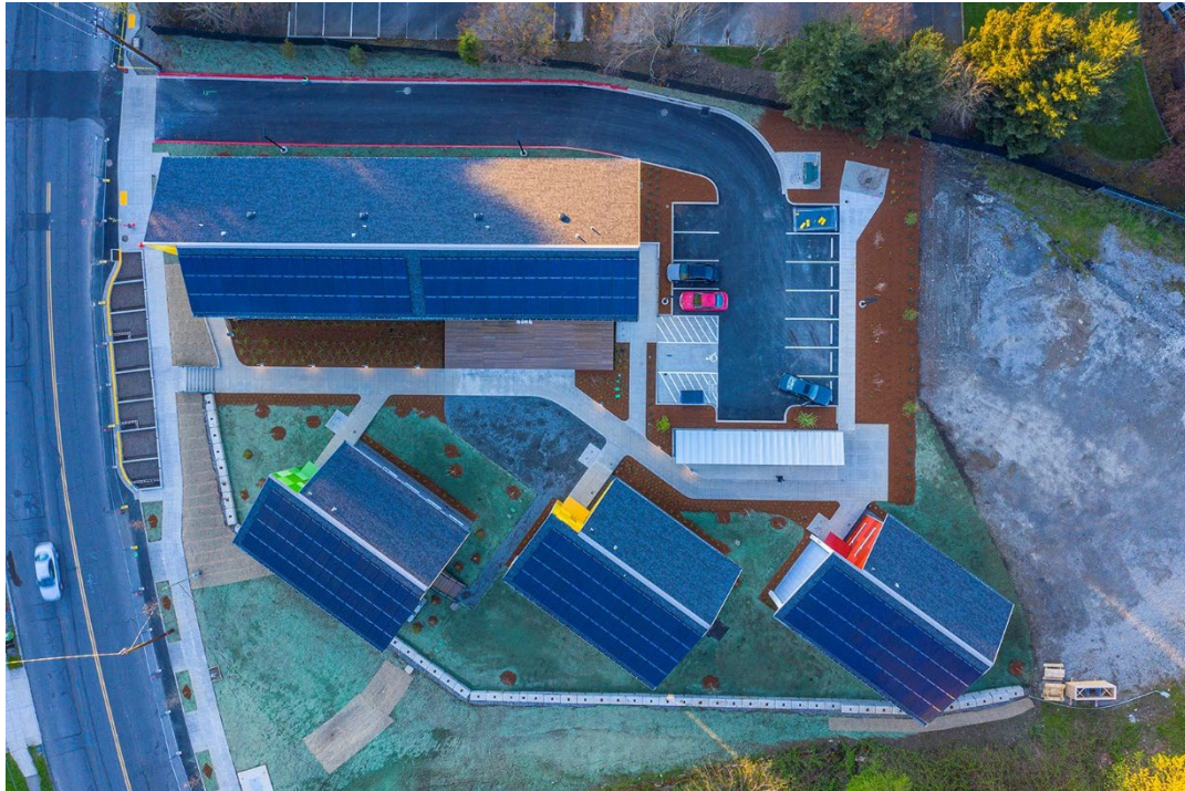
Figure 57. Image showing the layout of the site of Argyle Gardens. Credit: Holst Architecture
