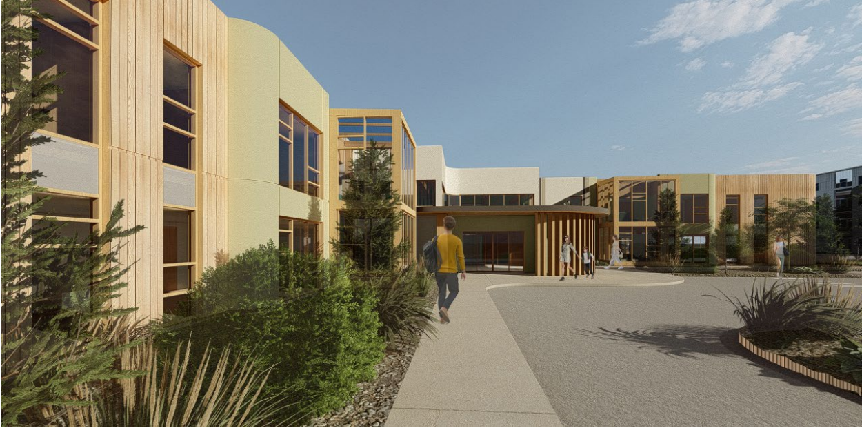
Figure 101. Exterior Perspective Walking Towards Main Entrance
