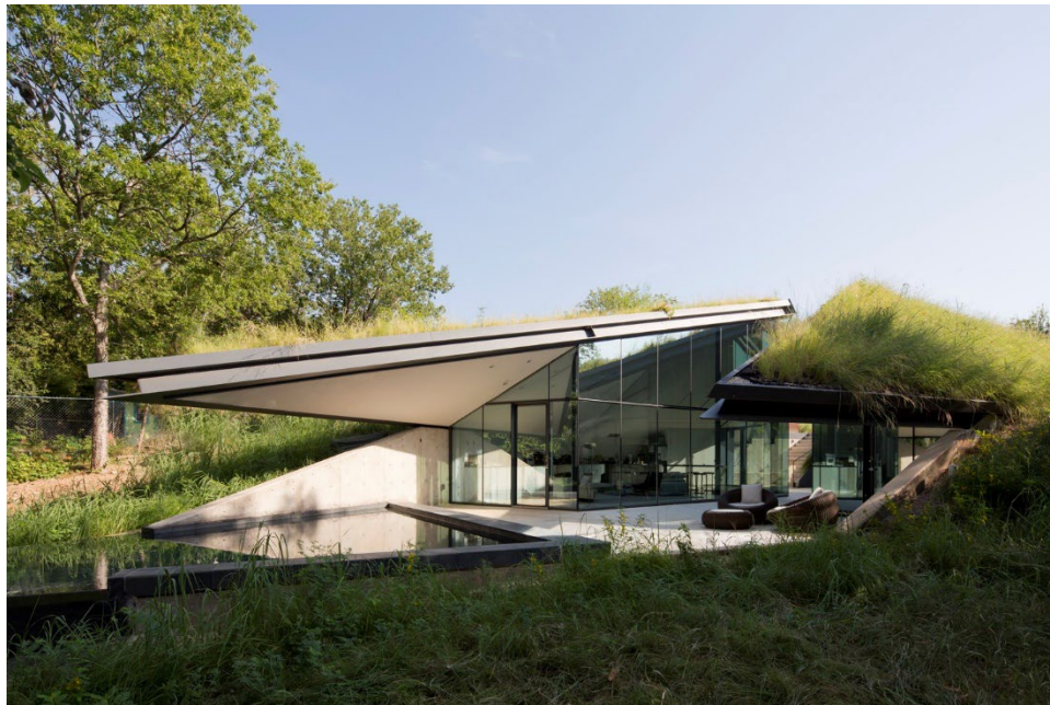
Figure 36. A picture the Edgeland house encompassed by earth
