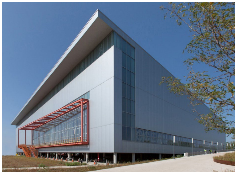
Figure 33. Ocean Breeze Track & Fieldhouse exterior view. This exterior view displays the raised aspect of the building to combat water from storm surges and high tides. Source: This figure was produced by Alexa Hoyer in Ocean Breeze Track & Fieldhouse / Sage and Coombe Architects, 2016 .
