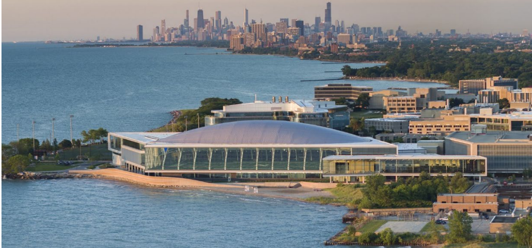
Figure 28. Ryan Fieldhouse and Walter Athletics Center north facing façade. Source: This figure was produced by James Steinkamp in Northwestern University Ryan – Walter Athletics Center / Perkins+Will, 2018 .
