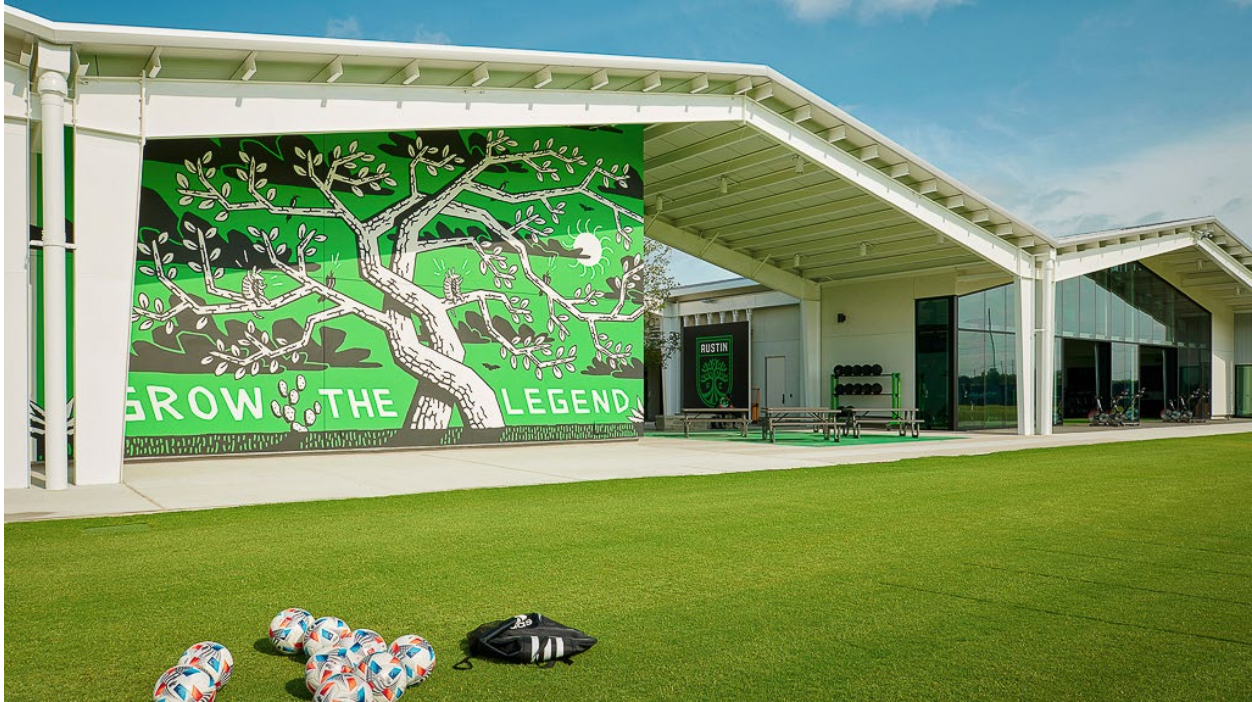
Figure 39. St. David's Performance Center Exterior view of St David's Performance Center. Source: This figure was produced by Gensler Architects in Designing performance centers to promote well-being for athletes, 2021 .
