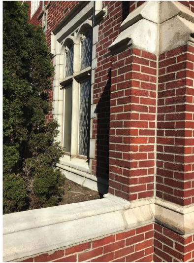
Precast concrete pilaster capitals and sills
