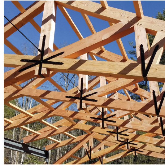
Heavy timber roof scissor trusses
