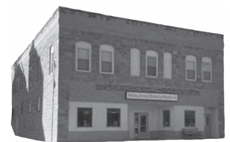
Current MUUS Block Building
