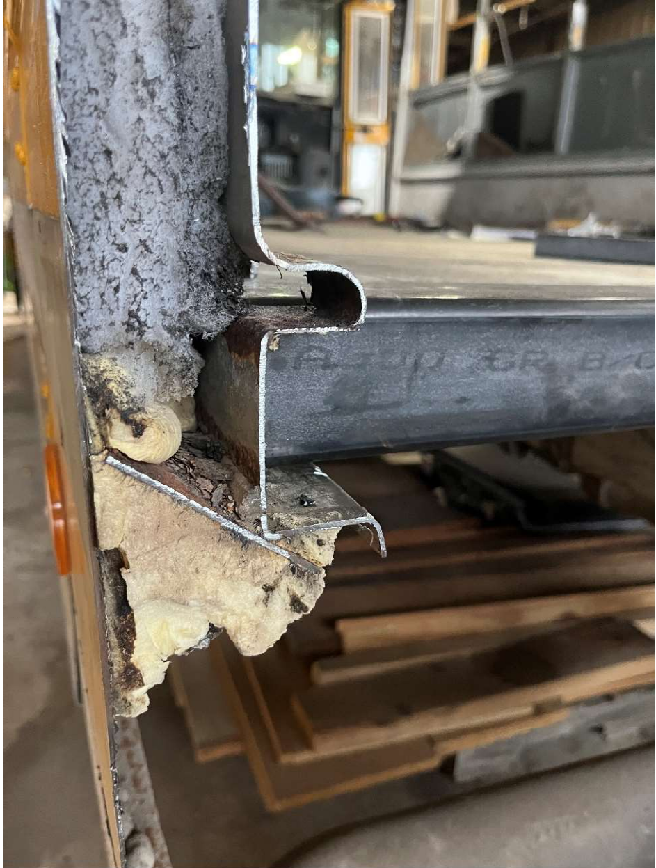
Figure 4.3.2.7 Steel tubing in Wall
