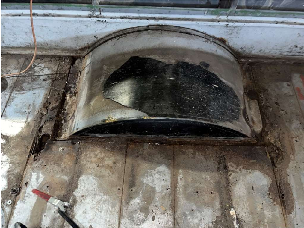
Figure 4.3.2.3 Wheel Well Existing
