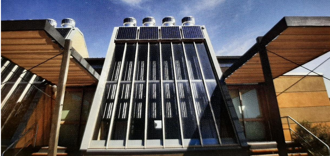
Figure 3.15. “Passive Ventilation System” (Ford, 2007)
