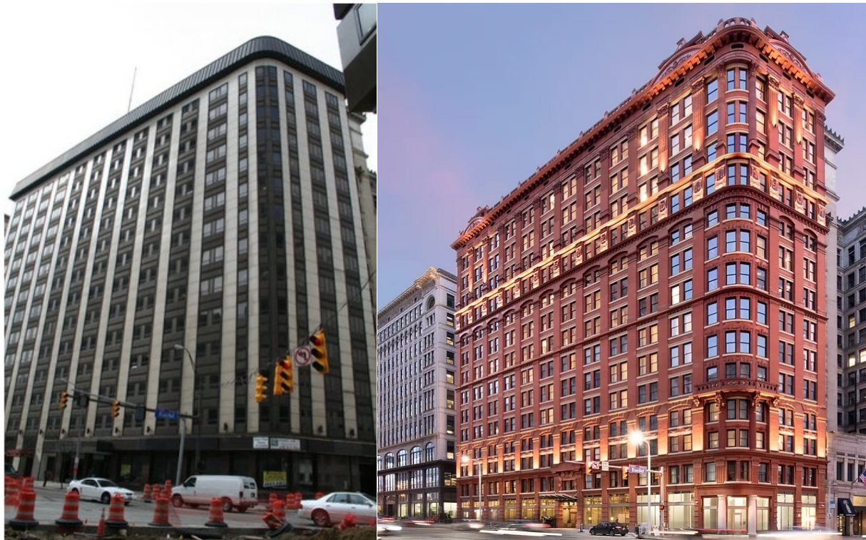
Figure 2.6, 2.7 The Schofield Building modernized 1960s (left) and restored 2016 (Right)
