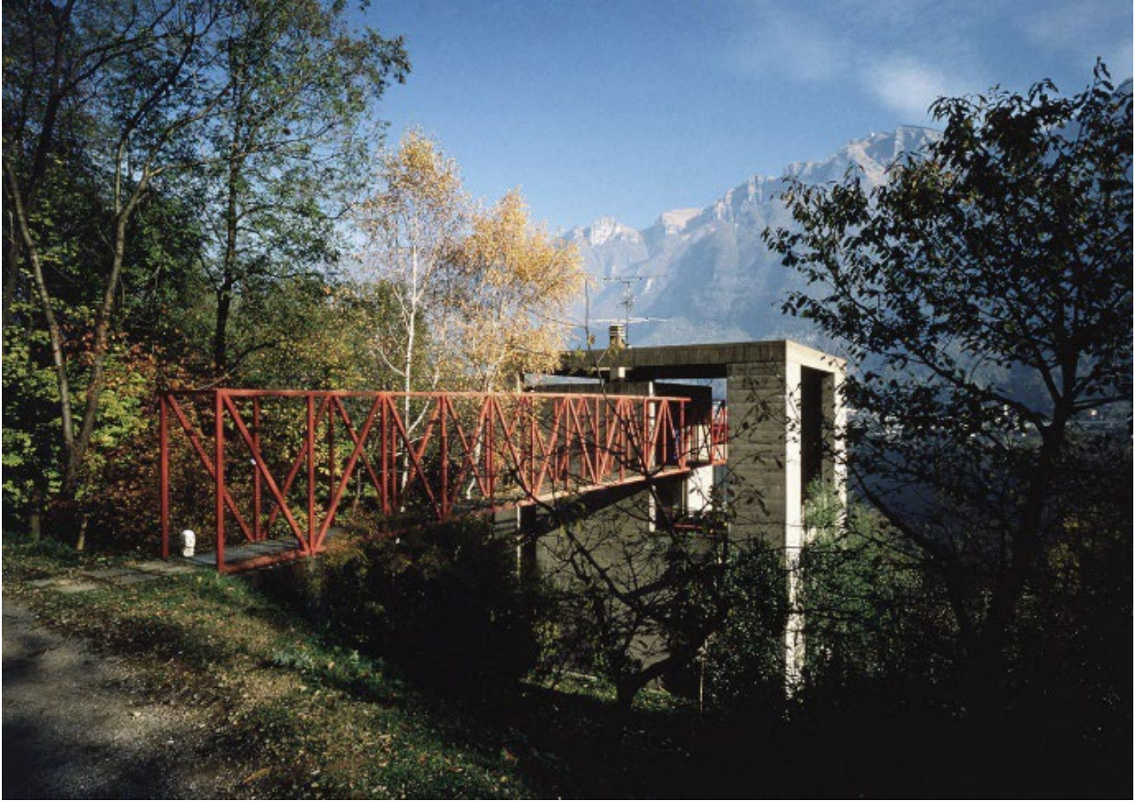
Figure 18 / Rear View of The Bianchi House
