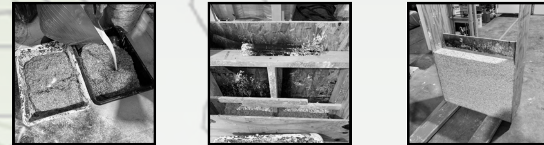
PREFABRICATED HEMPCRETE WALL PROCESS
