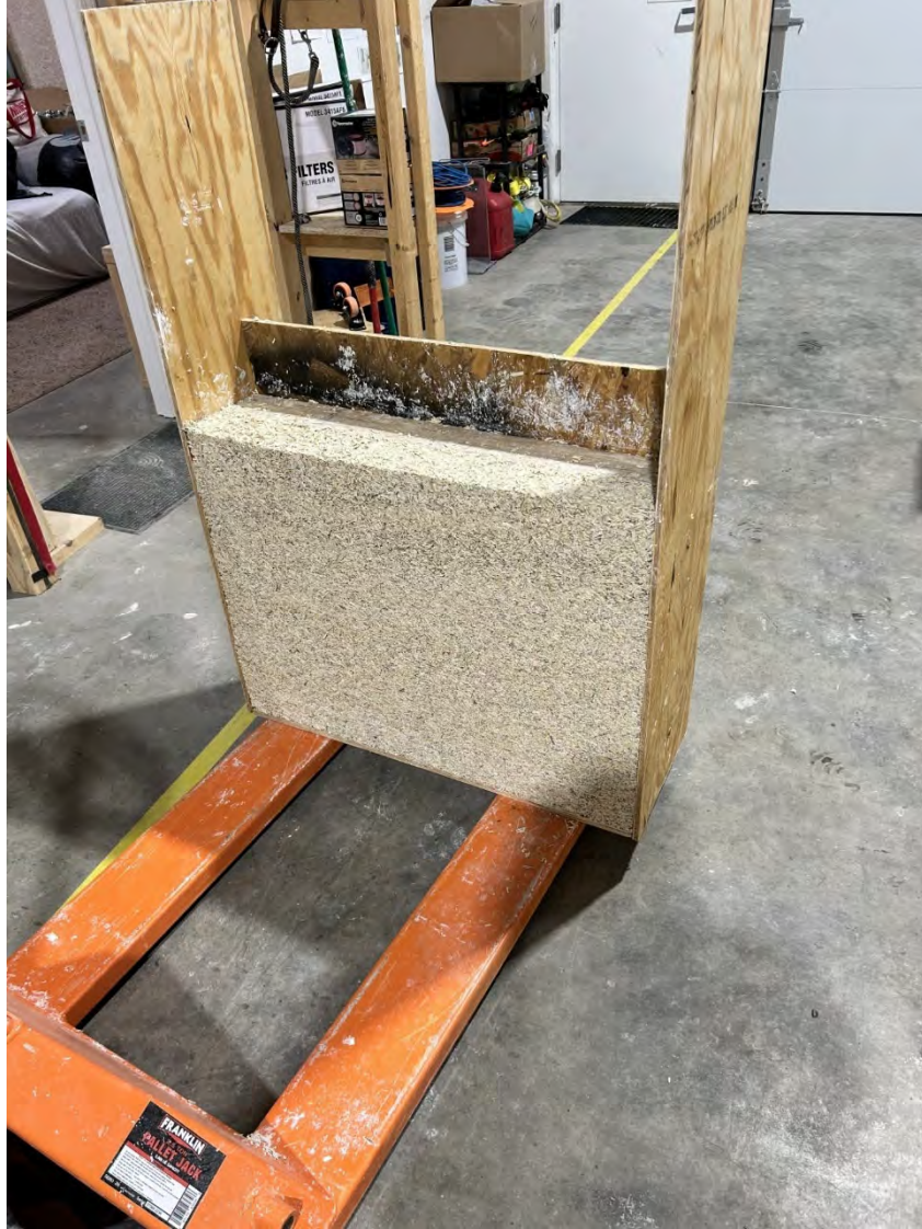
Figure 77. Finished Hempcrete Wall in Formwork
