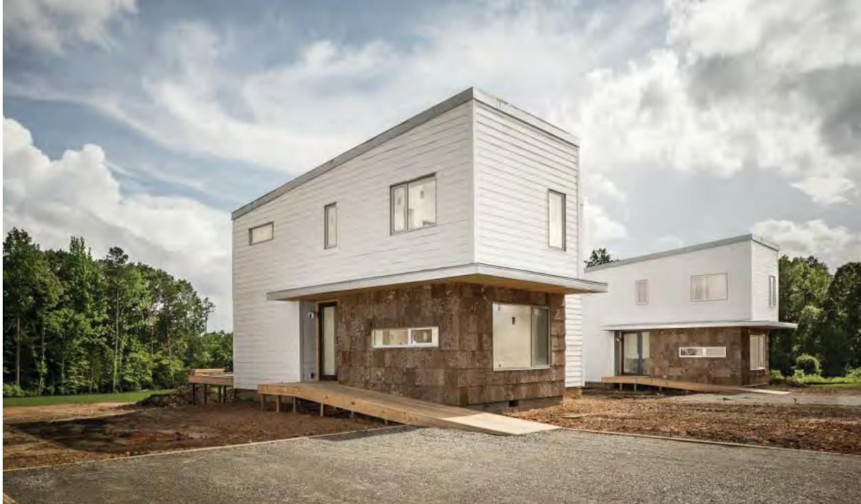
Figure 54. Prefab Passive House
