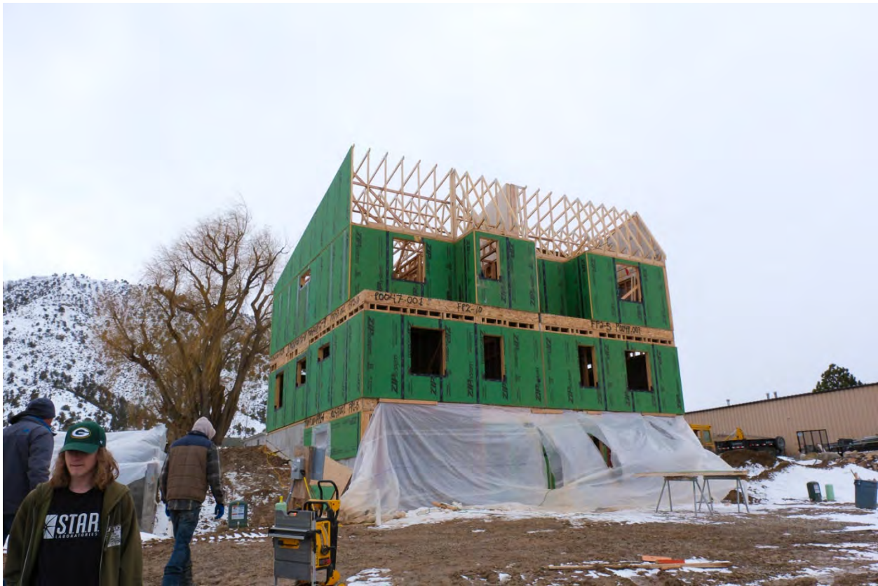
Figure 27. Affordable Housing Construction
