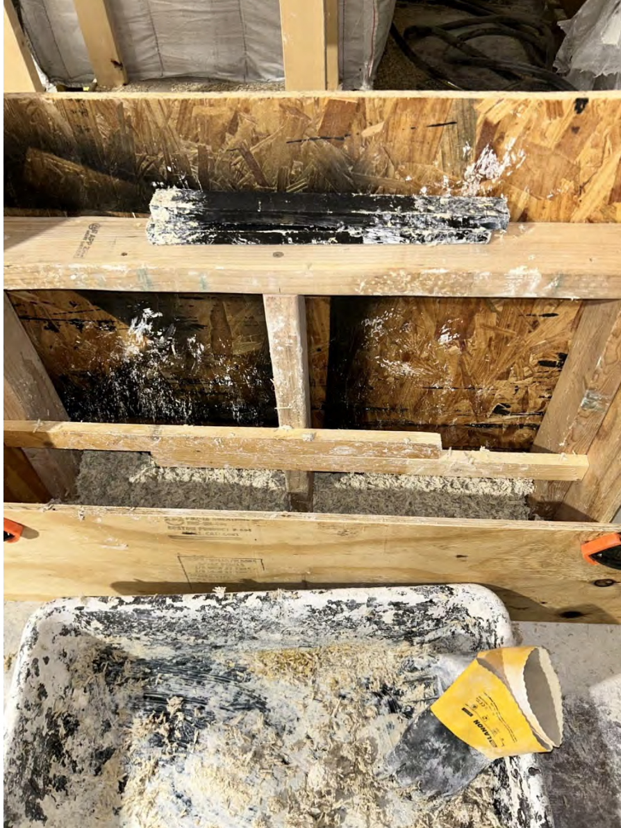
Figure 76. Partially Packed Hemp Wall
