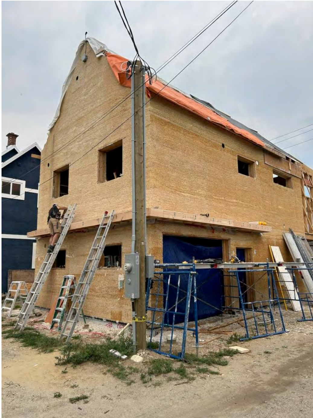
Figure 30. Two-Story Hempcrete House.
