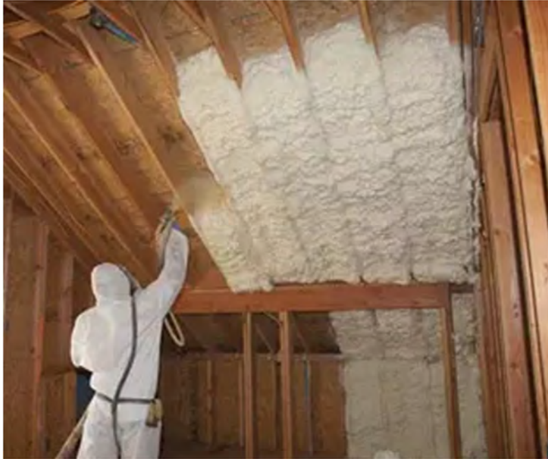
Figure 14. Spray Foam Insulation
