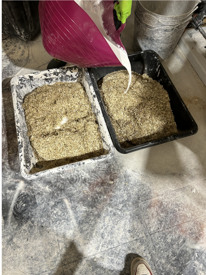
Hand mixing the lime and water in with the hemp shives.
