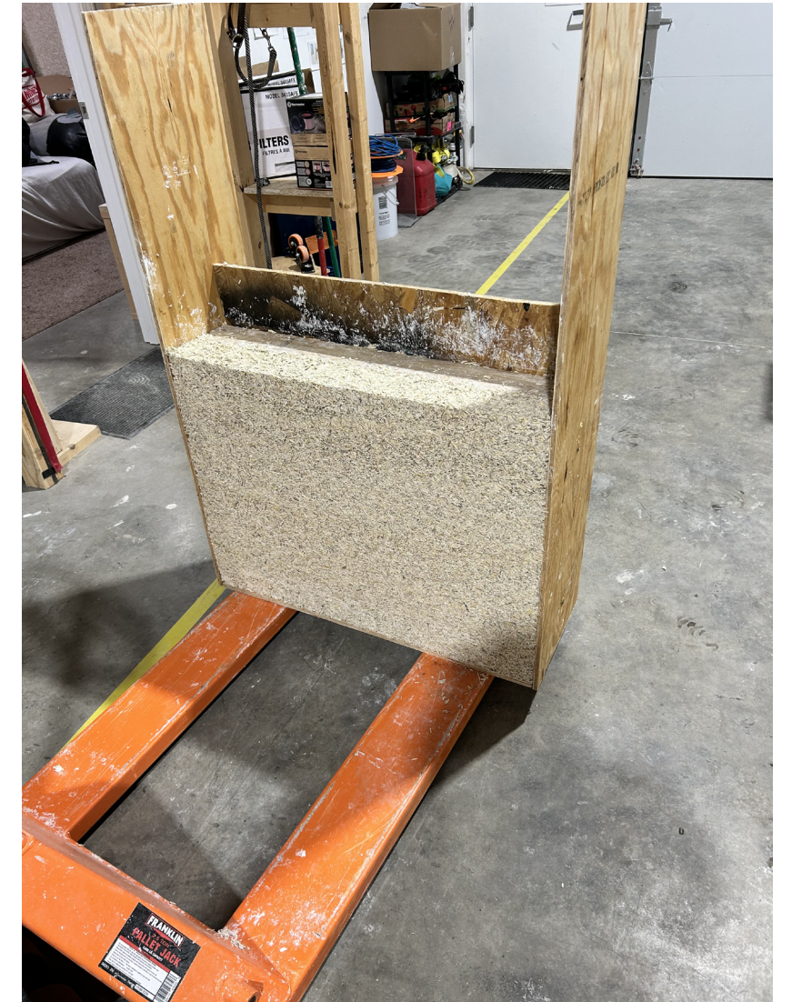
Remove formwork. Keep wrapped in plastic for 72 hours. Remove plastic and let set for 4-6 weeks so water evaporates completely.
