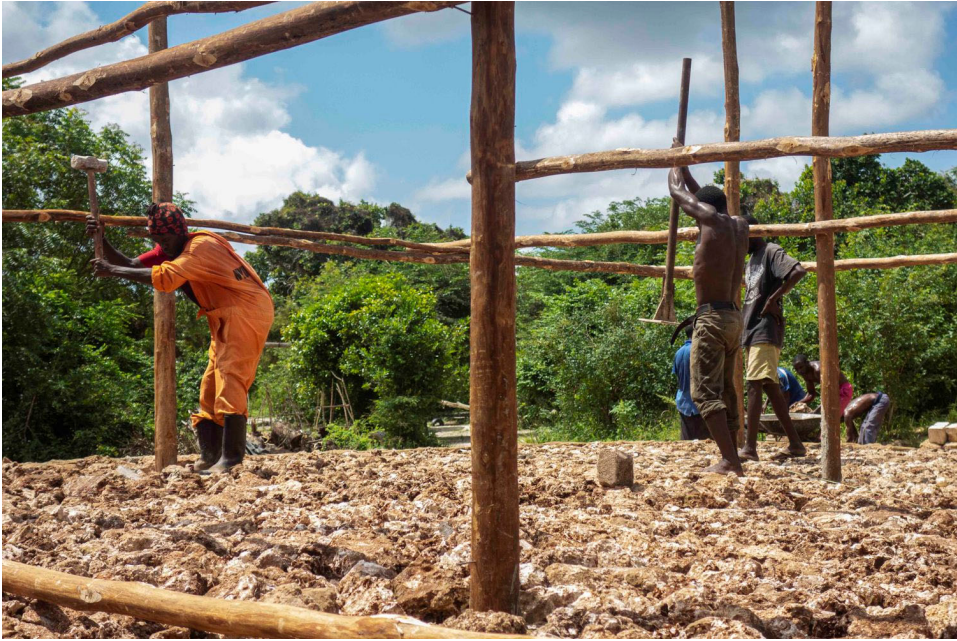
Figure 3.6.6.3 Construction of Eco Mayo Educational Centre (Caballero, 2020)
