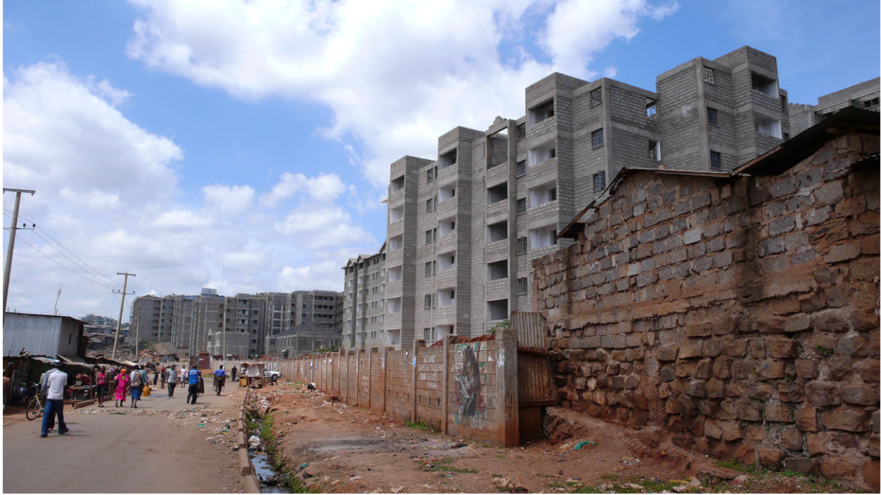
Figure 3.3.4 New Building Construction in Kibera (Google)
