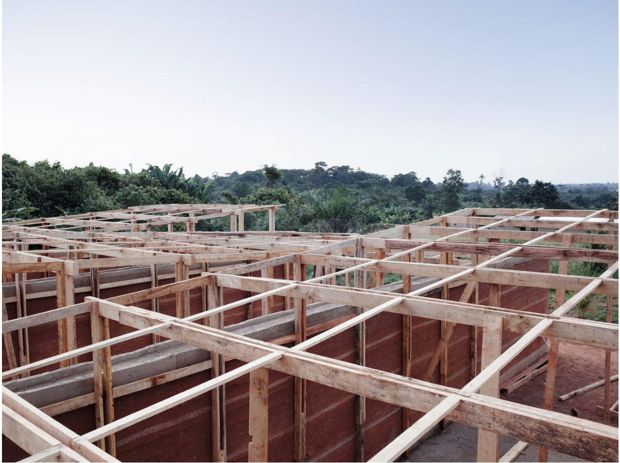
Figure 3.6.4.3 Photo During the Construction of InsideOut School (Tapia, 2020)
